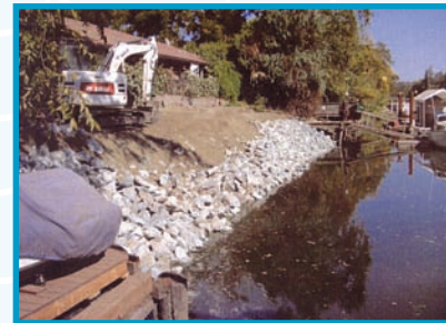
New riprap on levee
