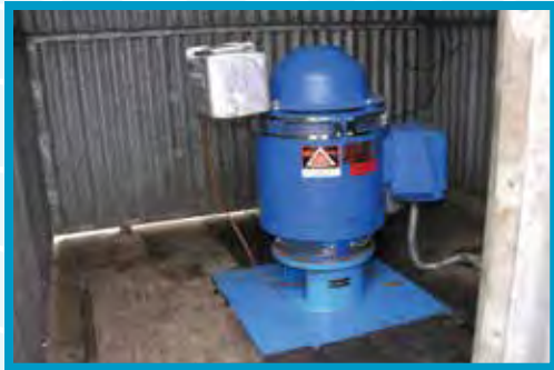
Pump Station No. 10 Hogue Avenue/Tyler School-discharge pump
