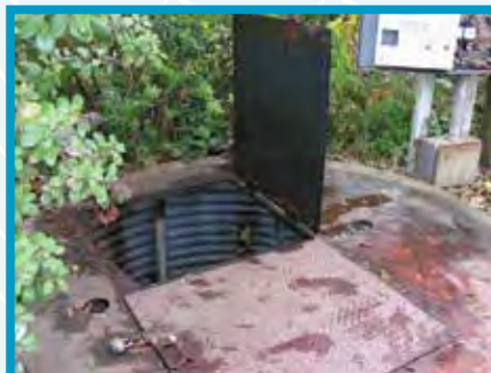
Pump Station No. 6 Moreing Road-new secure steel sump cover
