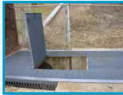
Pump Station No. 8 Kirk Avenue-new steel grating with access door for debris removal
