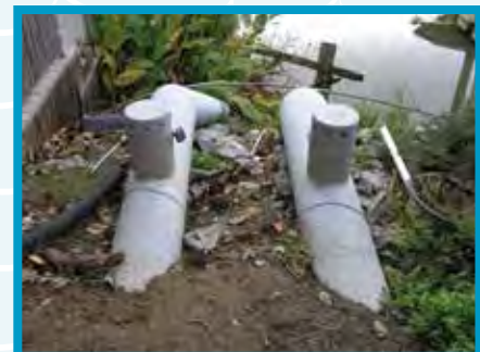
Pump Station No. 5 Gardena- new siphon relief valve seals
