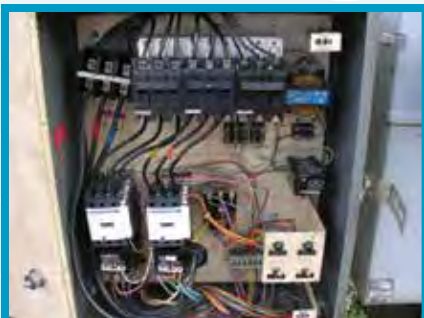
Pump Station No. 6 Moreing Road-new circuit breakers for discharge pump 6W
