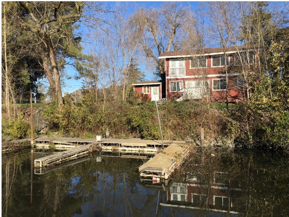
2011 Mission Rd.: A more easily inspectable property with a dock in disrepair.
