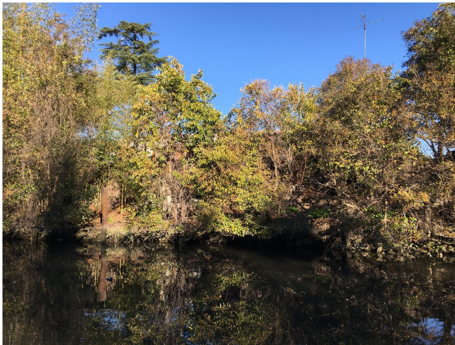
1448 W.S. Tuxedo Ave: Dense vegetation renders the waterside slope invisible.
