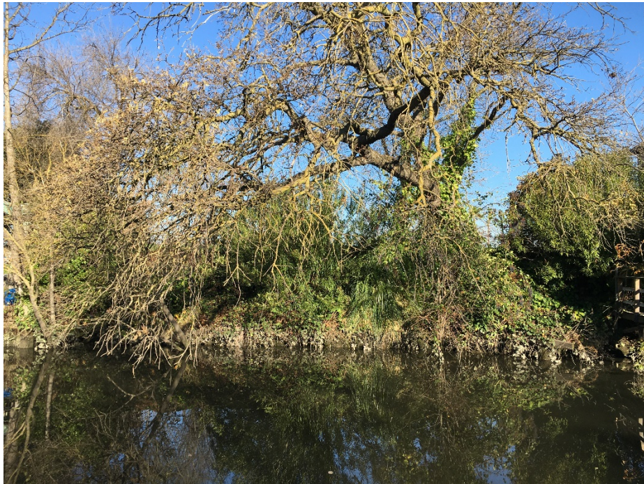
1534 W.S. Tuxedo Ave.: A large tree overhanging the canal coupled with lots of dense vegetation render the waterside slope uninspectable.
