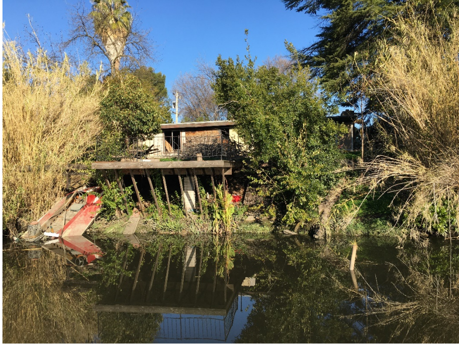
1848 W.S. Tuxedo Ave.: A burned-out home surrounded by dense vegetation provides zero inspectability of the waterside slope.
