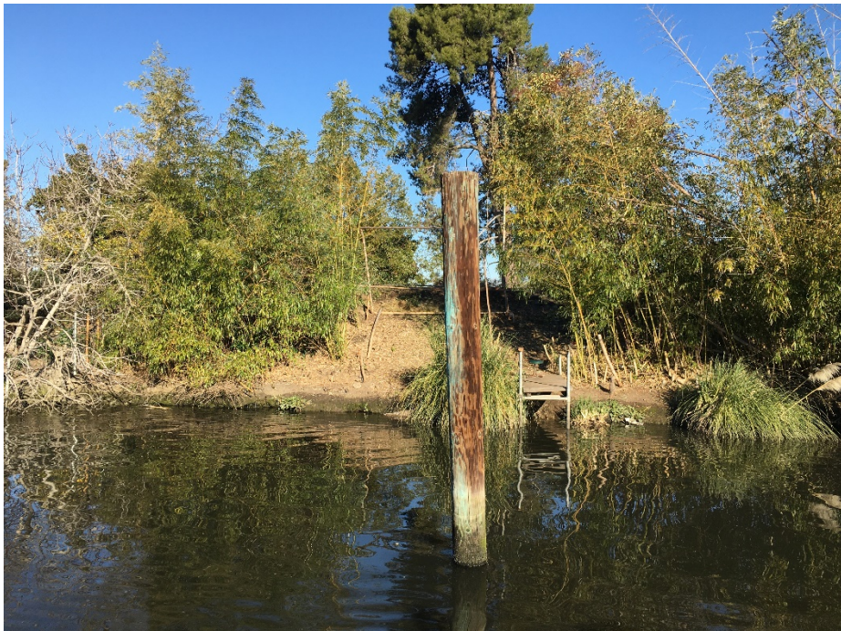
2060 Canal Dr.: Dense vegetation comprised of fast-growing bamboo render this slope uninspectable most of the time. Sometimes someone cuts it near the dilapidated dock.
