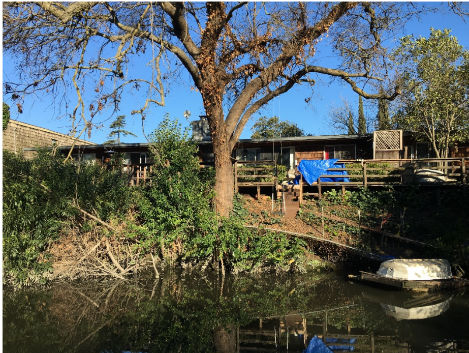
1640 W.S. Tuxedo Ave.: Large tree, dense vegetation, and dock in disrepair.
