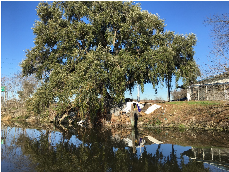
2020 Plymouth Rd.: Another prime candidate for rock slope protection, although an illegal camper has constructed a ramshackle home on the waterside slope.
