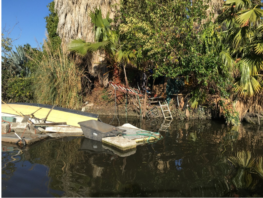
2260 Via Milano Pl.: Dense vegetation provides ample protection from the elements for an illegal camper. The thick vegetation also prevents inspectability of the waterside slope and the sunken boats create a navigation hazard in the canal.
