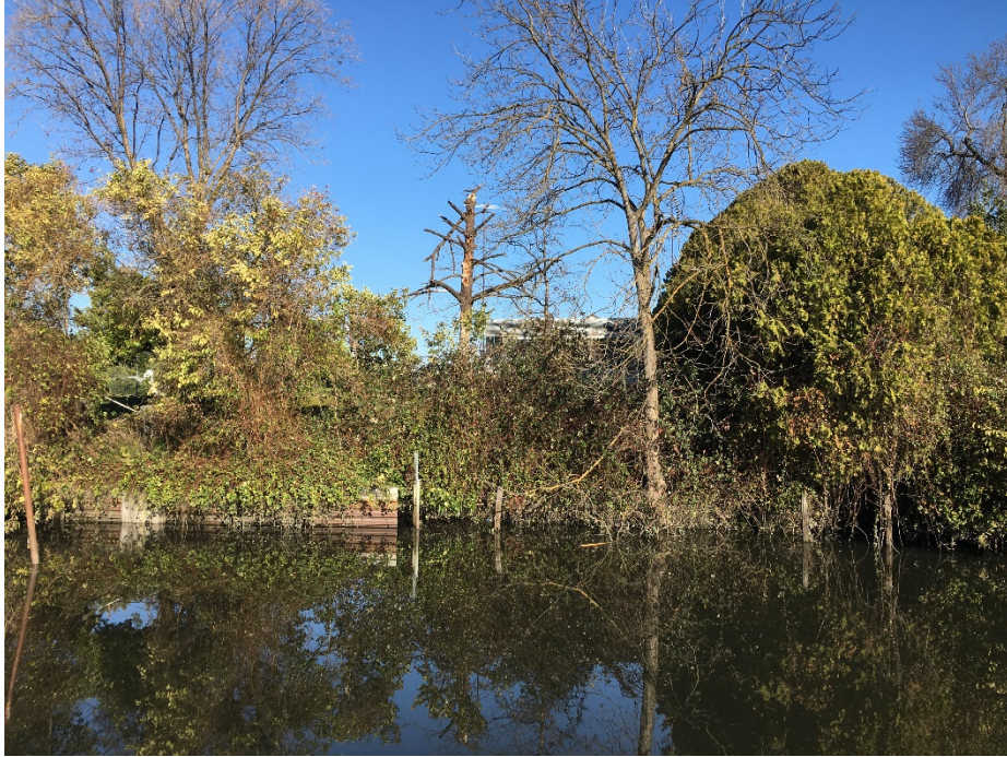
1948 Canal Dr.: Dense vegetation coupled with a metal 'headwall' provides zero inspectability along the waterside slope.
