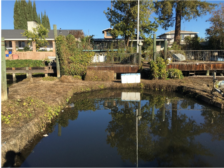
2344 Canal Dr.: This is what happens to rickety docks left in place by the property owners.
