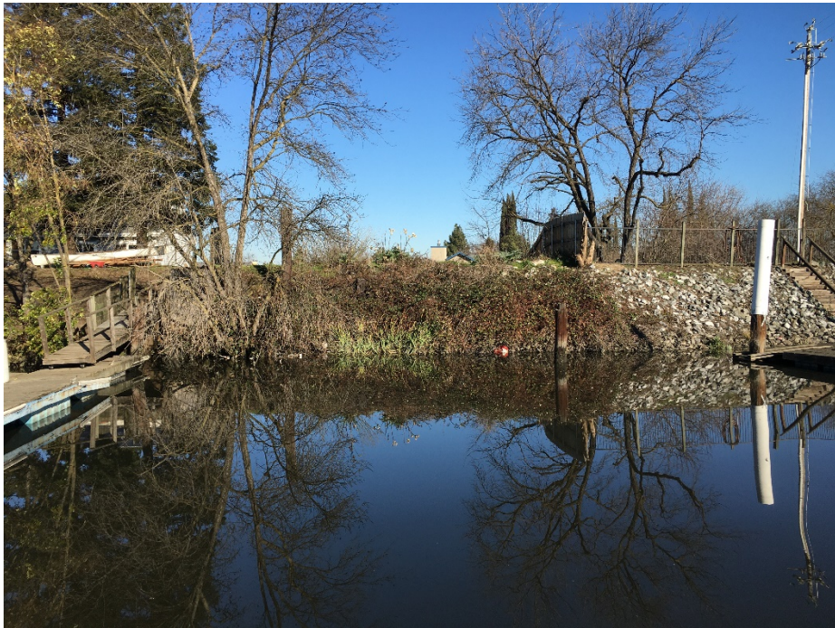
2204 Canal Dr.: A good candidate for riprap.
