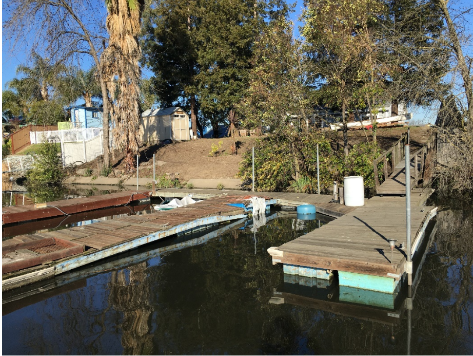
2220 Canal Dr.: This homeowner has verbally agreed with the District for rock slope protection.
