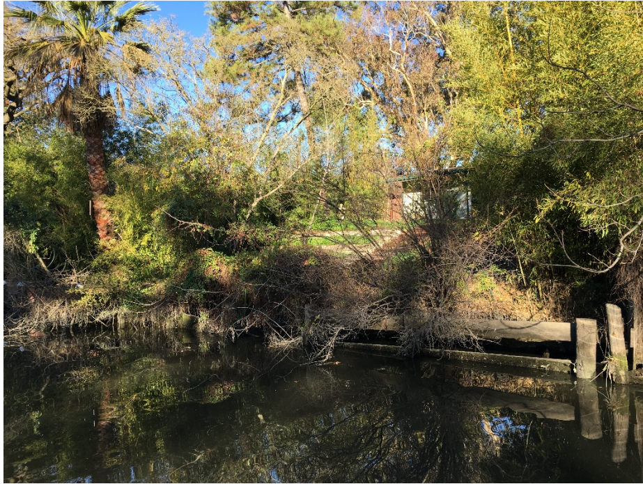
1466 W.S. Tuxedo Ave: Wooden 'headwall' and dense vegetation.
