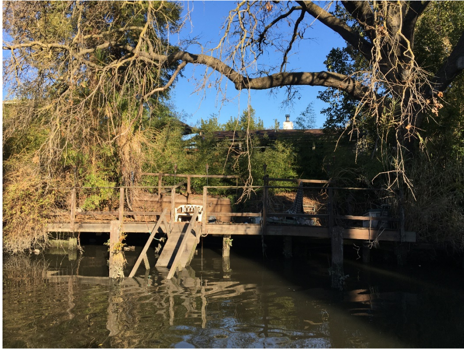
1510 West South Tuxedo Ave.: Dense vegetation and a deck in a state of disrepair.
