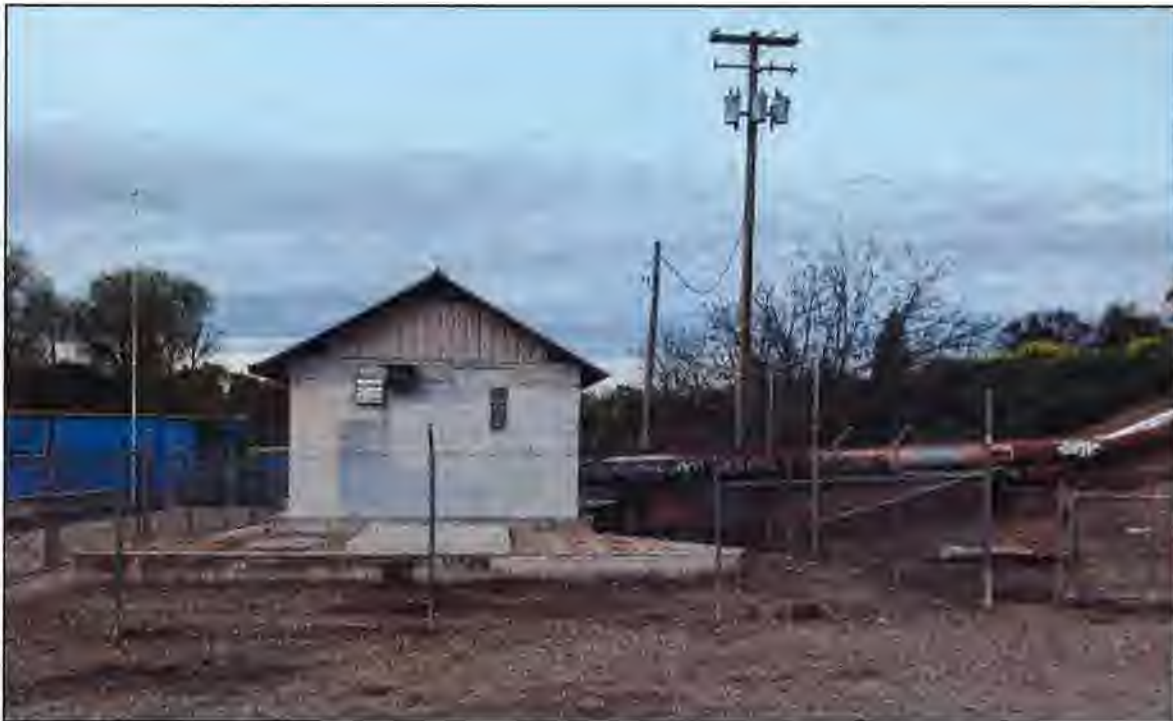
Photograph 1. Wisconsin Pump Station - view to West
