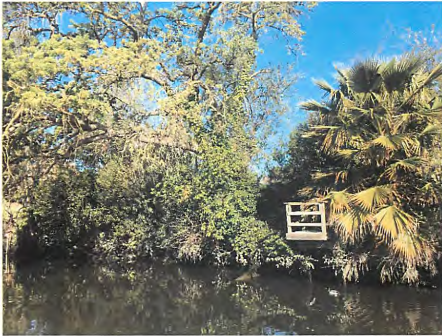
1534 W. S. Tuxedo Ave.: Another dilapidated dock and dense vegetation overhanging the canal.
