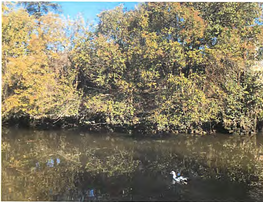
1448 W. South Tuxedo Ave.: Excess vegetation encroaches into the canal.
