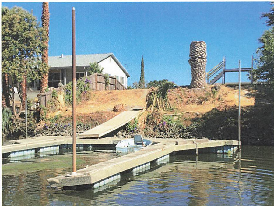
2038 Canal Drive: The waterside slope is bare and riprap-ready if the homeowner desires.
