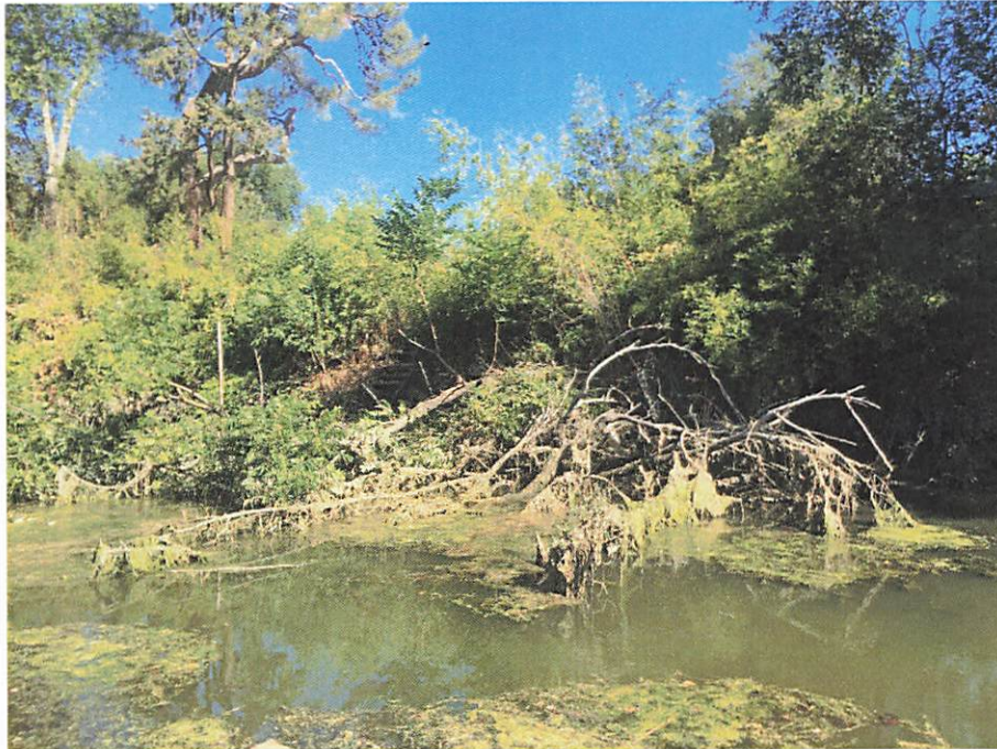
1842 W. S. Tuxedo Ave.: Some trimming from homeowner is evident and trees have fallen into the canal.
