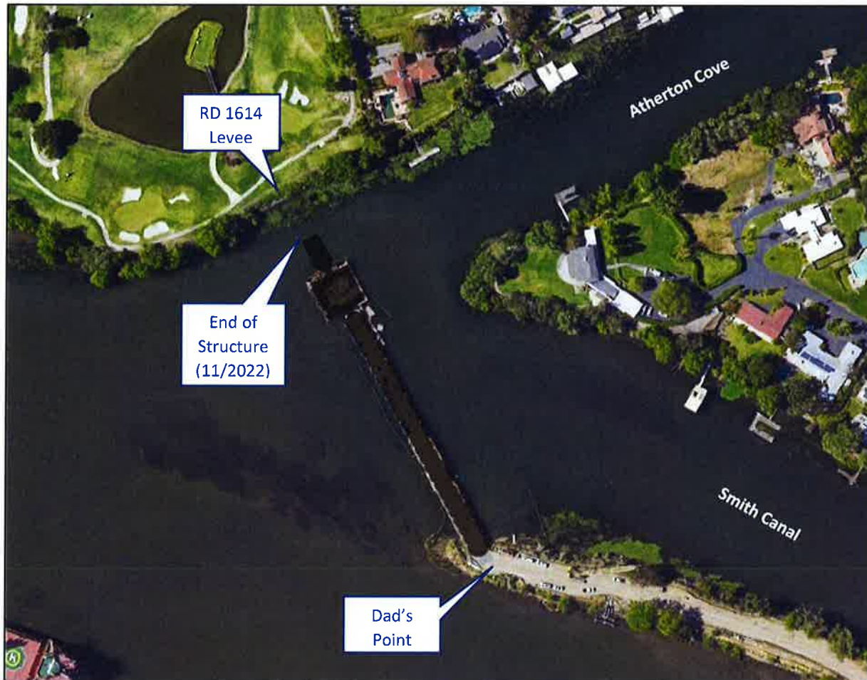
Figure 1. Current Construction Status of Smith Canal Gate Project
