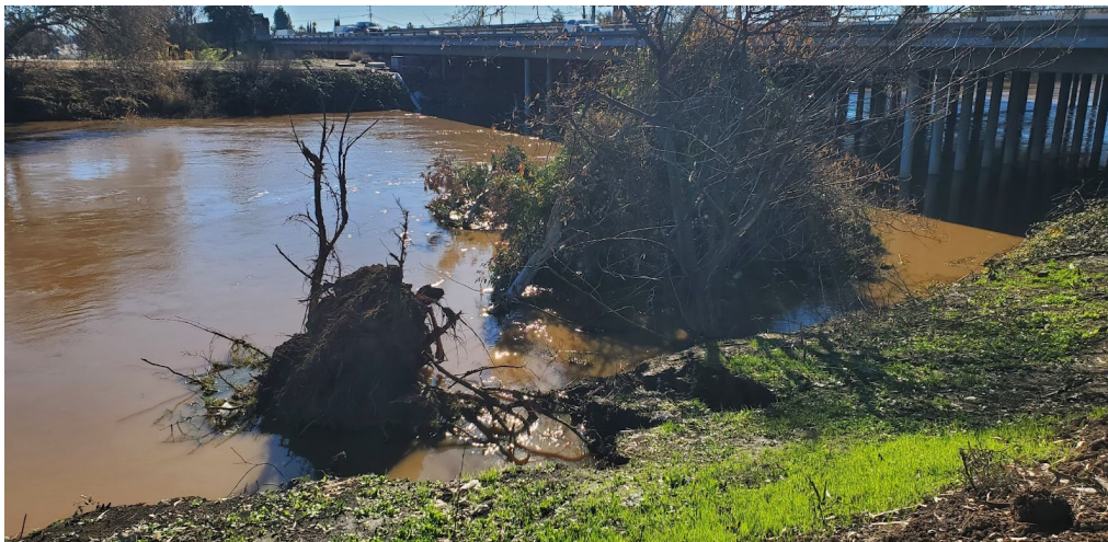
Big tree on levee at north shore calaveras river and I/5 - a large section of levee was washed away. SJ C Channel maintenance removed the tree and began emergency repair work.
