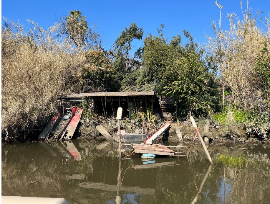
1848 W S Tuxedo Avenue: This home is on the City of Stockton's demolition list for this year. During January's storm event, a large tree fell on the house, rendering it more qualified for demolition.
