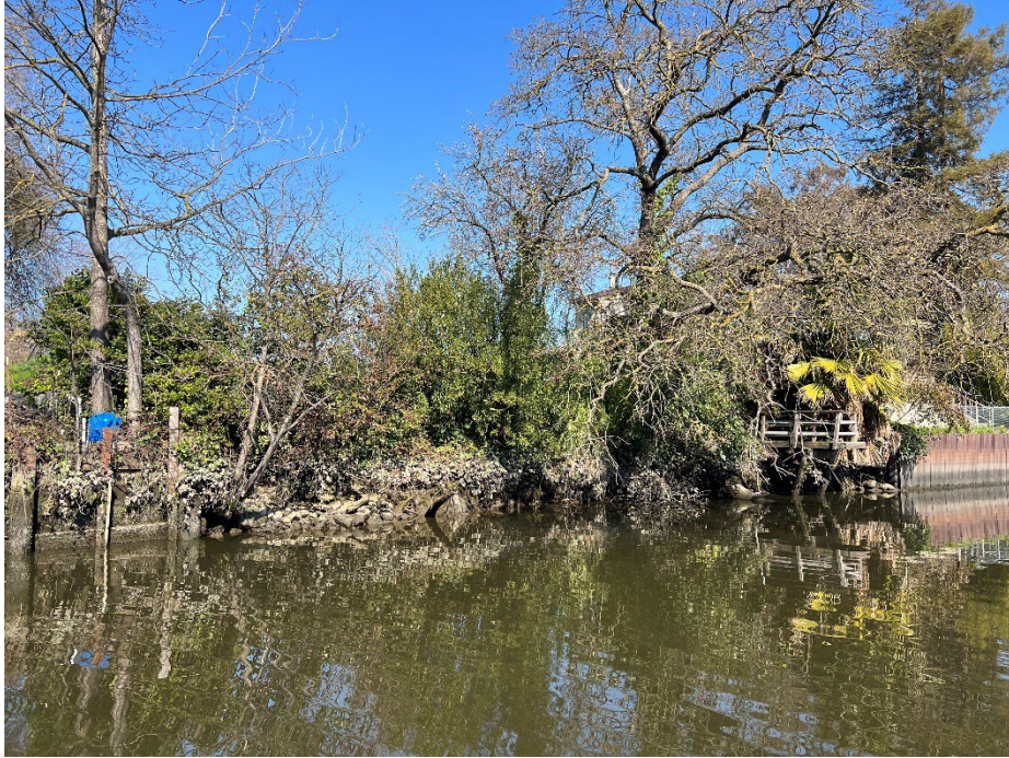
1534 W S Tuxedo Avenue: Dense waterside vegetation renders inspection of the slope impossible.
