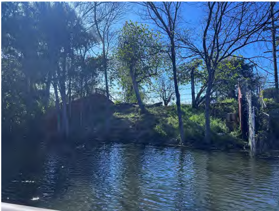
1775 Walnut St.: No rock on waterside slope.
