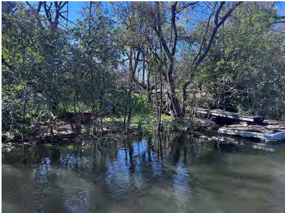
1855 W. Harding Way: More dilapidated docks and debris piles beneath dense vegetation on the waterside slope.
