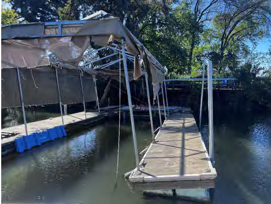
1733 Walnut St.: Dock sits unused for many years and no rock on waterside slope.
