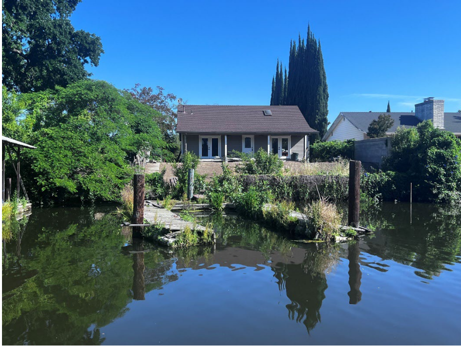
2364 Canal Drive: This property will be receiving RSP in the upcoming maintenance year.
