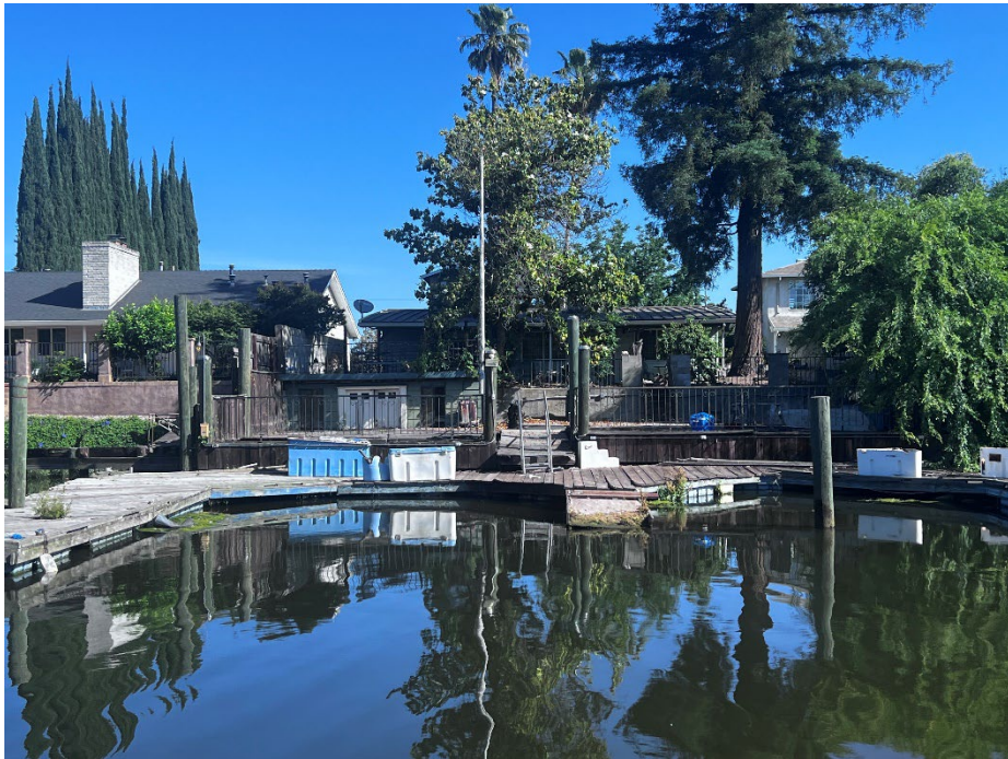
2344 Canal Drive: Dilapidated docks with no boat seen in years.
