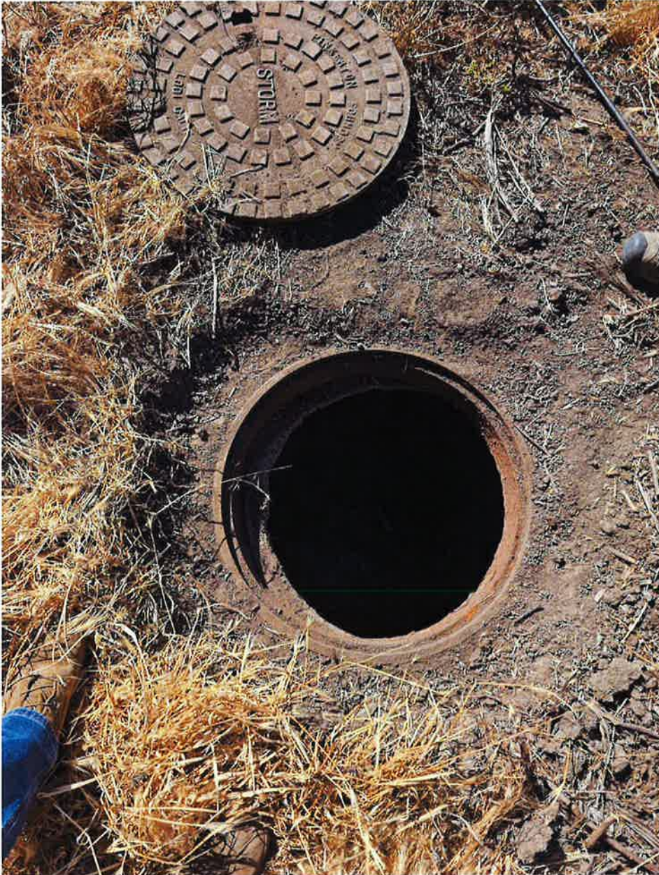
MH-3 Figure 4: Condition of MH-3.
