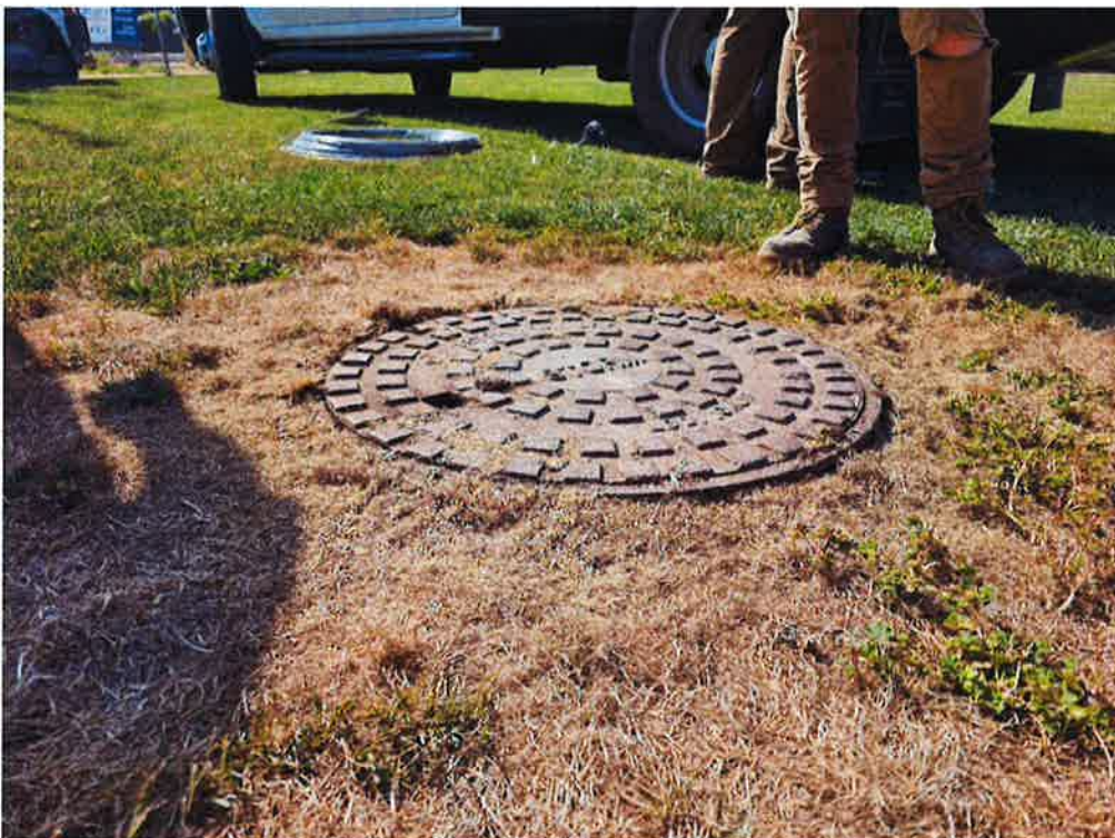
MH-5 Figure 4: Condition of MH-5.
