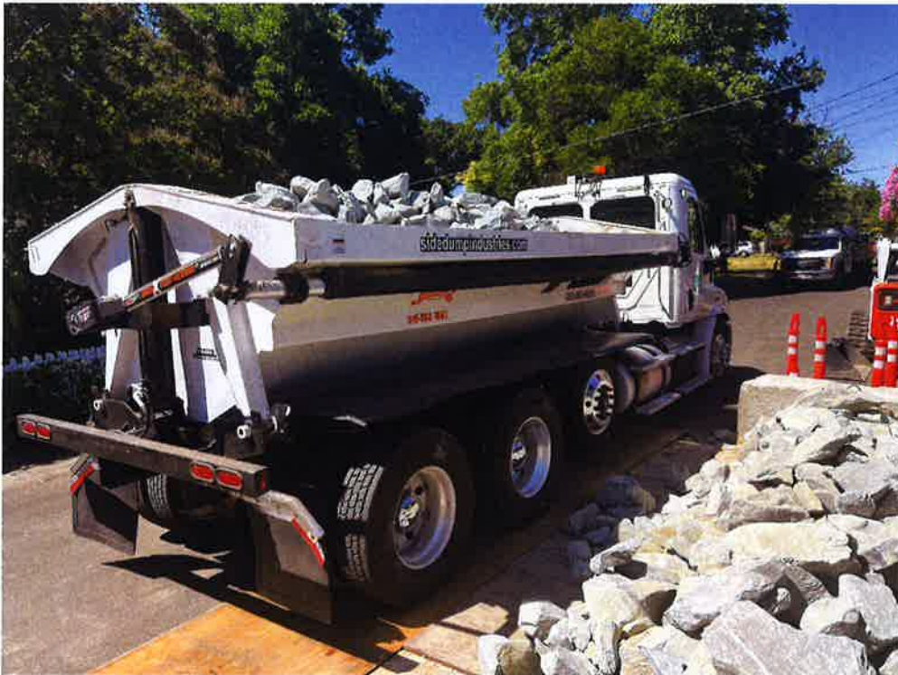
1968 Canal Drive: A 15' trailer dumps 18" minus rock into a protective barrier.
