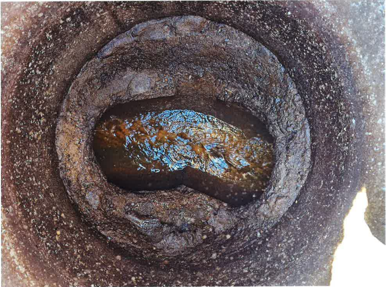
MH-5 Figure 6: Condition of MH-5.
