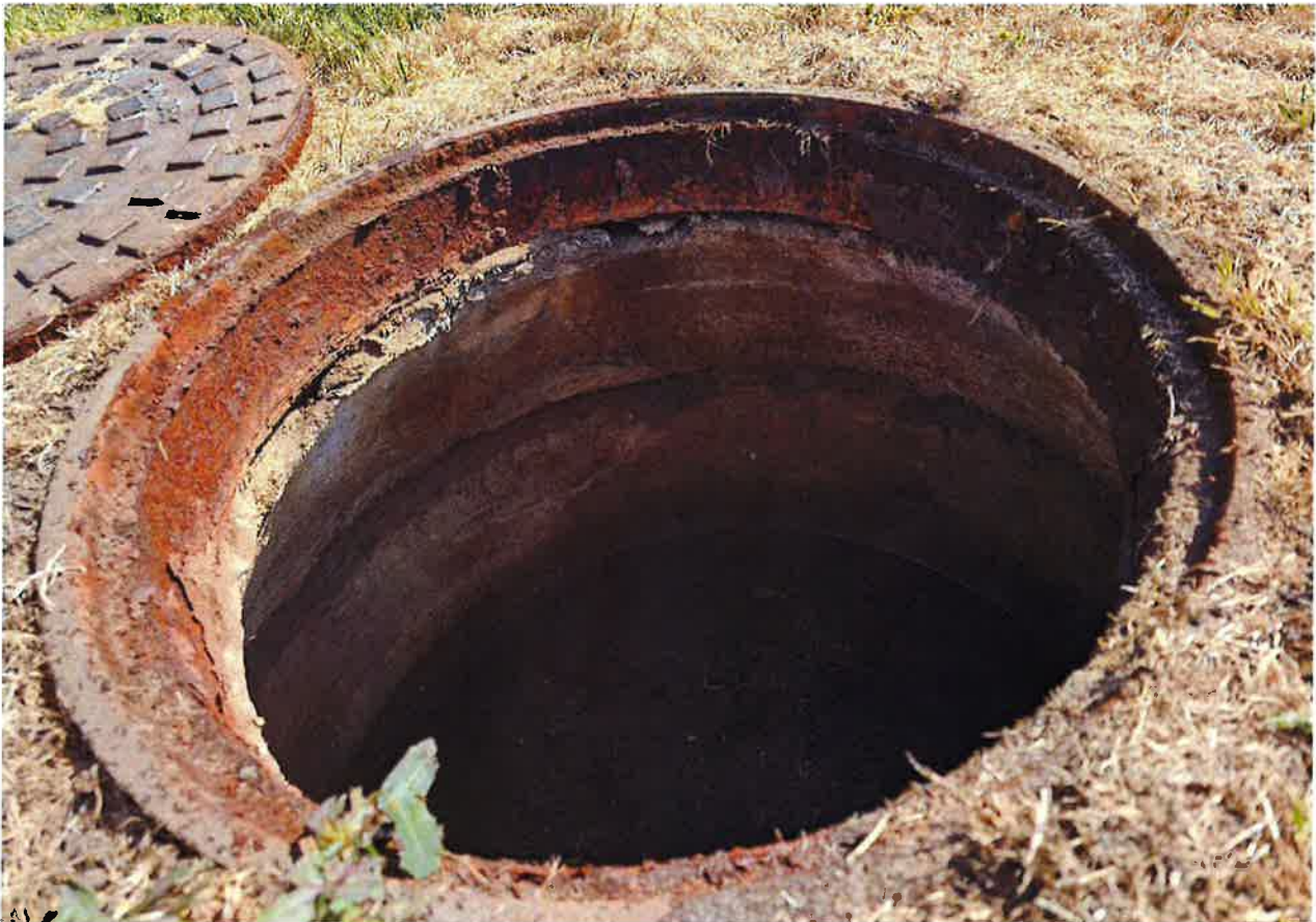
MH-4 Figure 5: Condition of MH-4.
