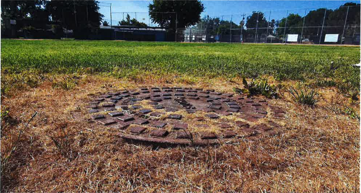
MH-4 Figure 4: Condition of MH-4.
