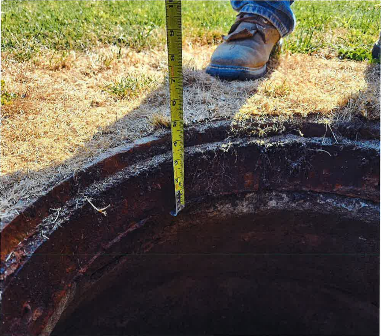
MH-5 Figure 5: Condition of MH-5.
