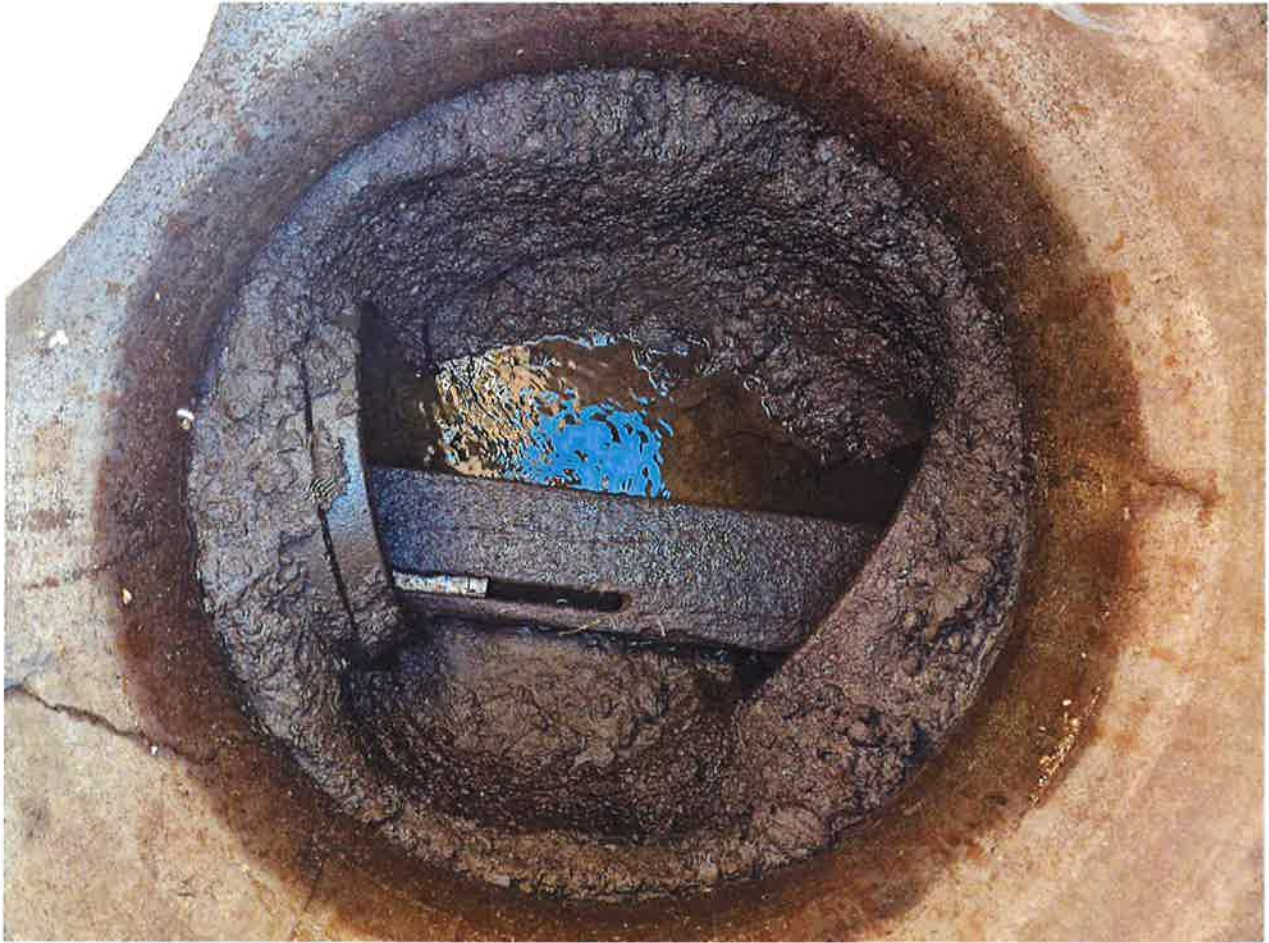
MH-4 Figure 7: Condition of MH-4.
