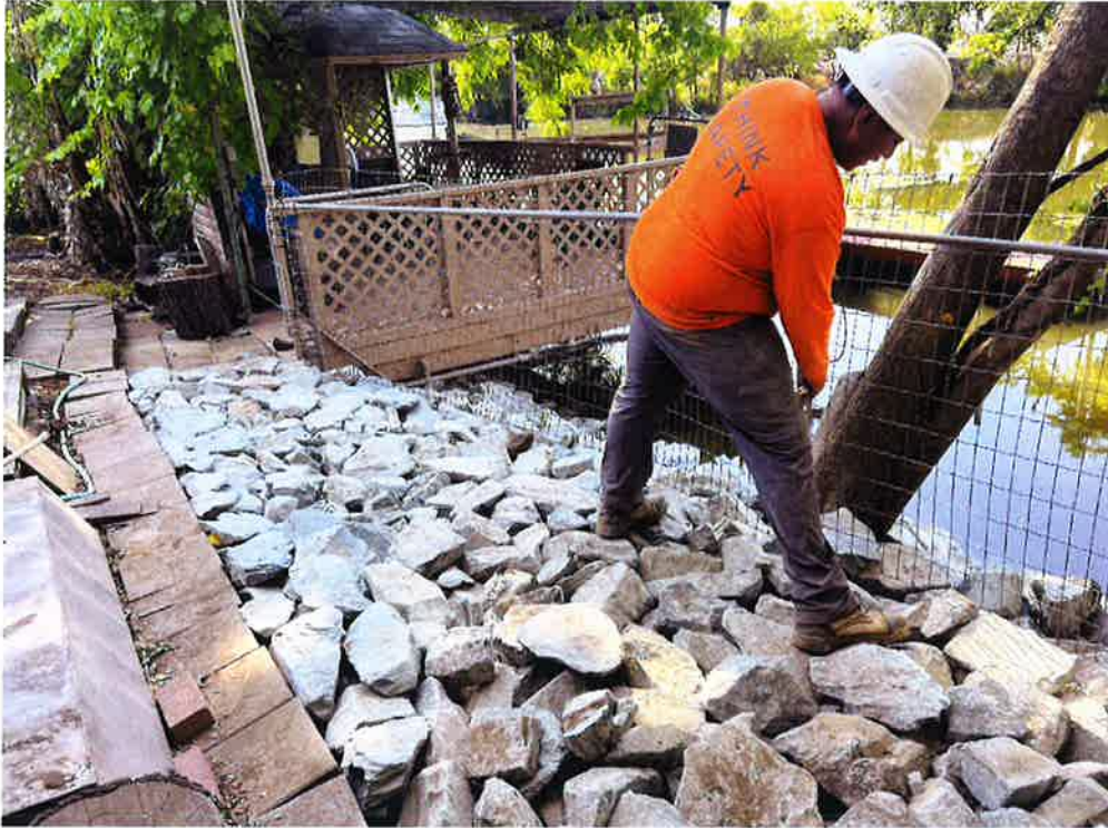
1960 Canal Drive: Laborers replace the waterside fence after RSP placement.
