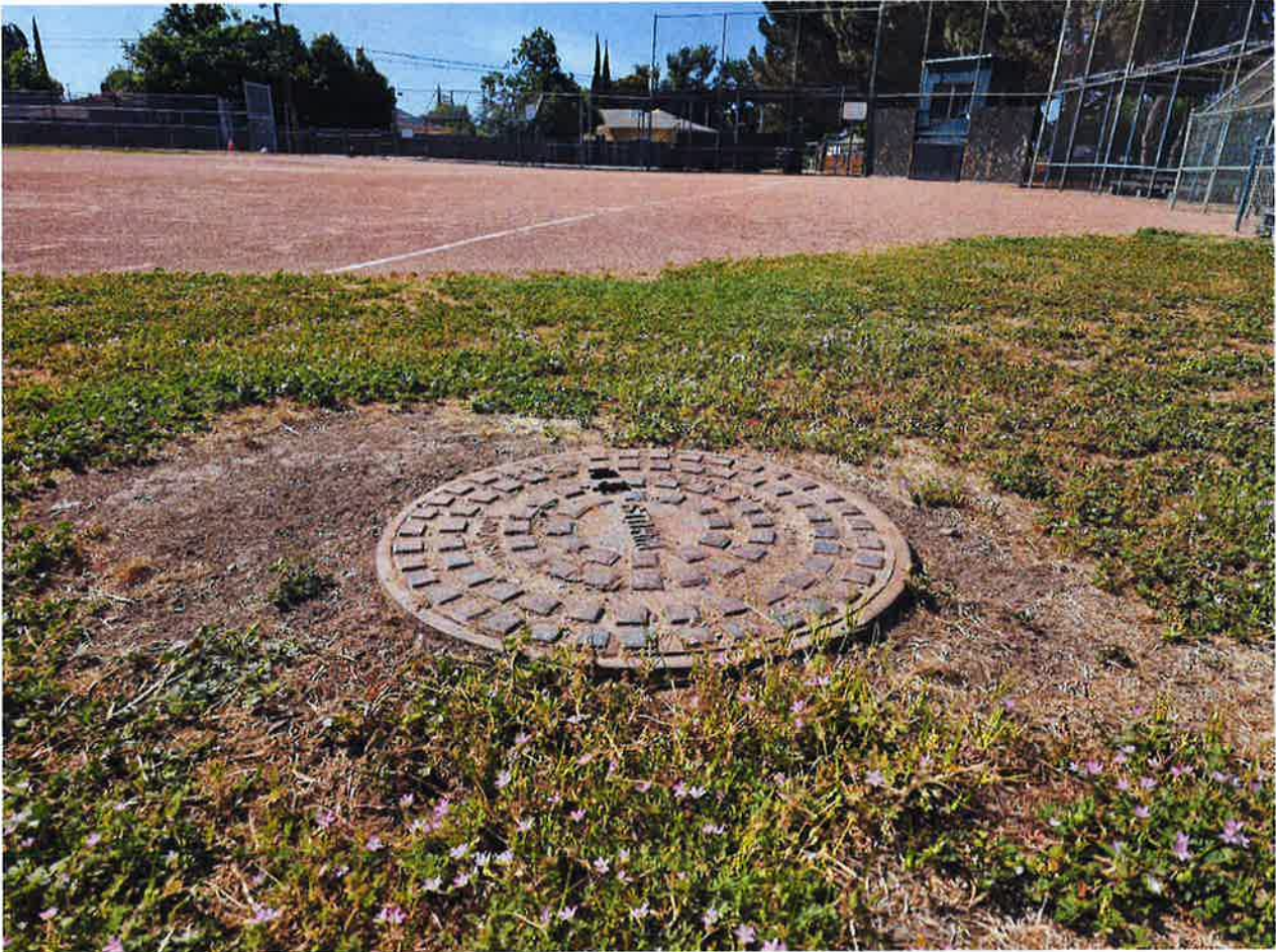
MH-2 Figure 7: Condition of MH-2 facing south-west.
