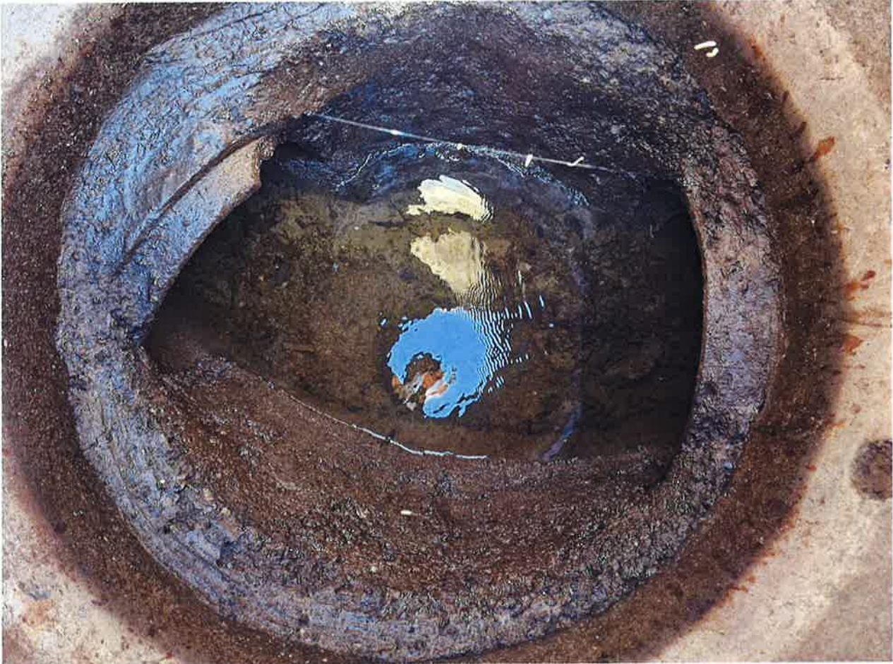
MH-2 Figure 8: Condition of MH-2.
