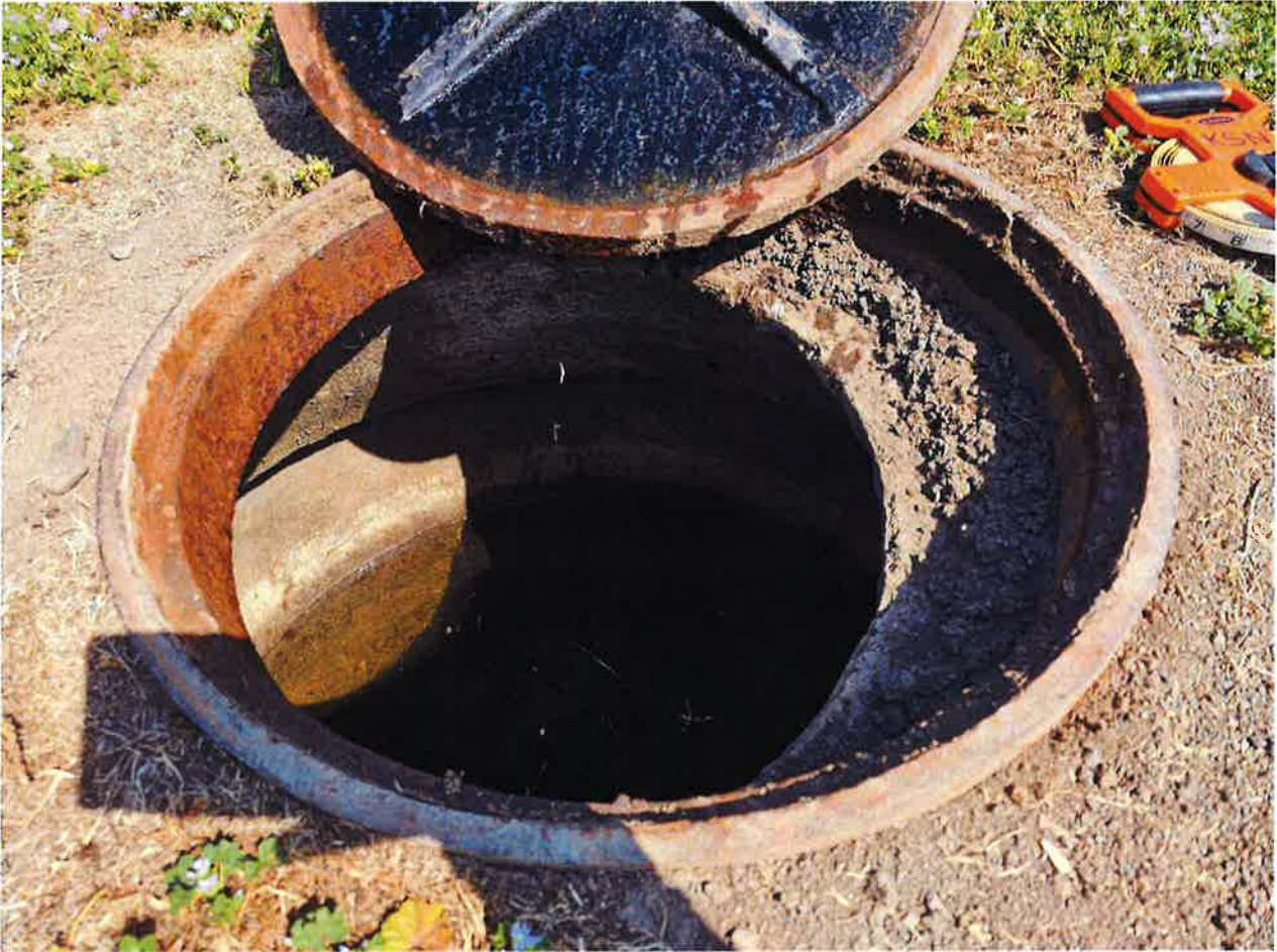
MH-2 Figure 5: Condition of MH-2.
