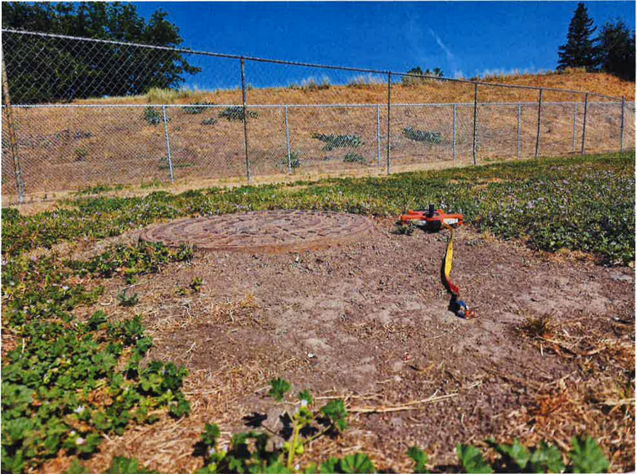
MH-2 Figure 6: Condition of MH-2 facing levee (north).
