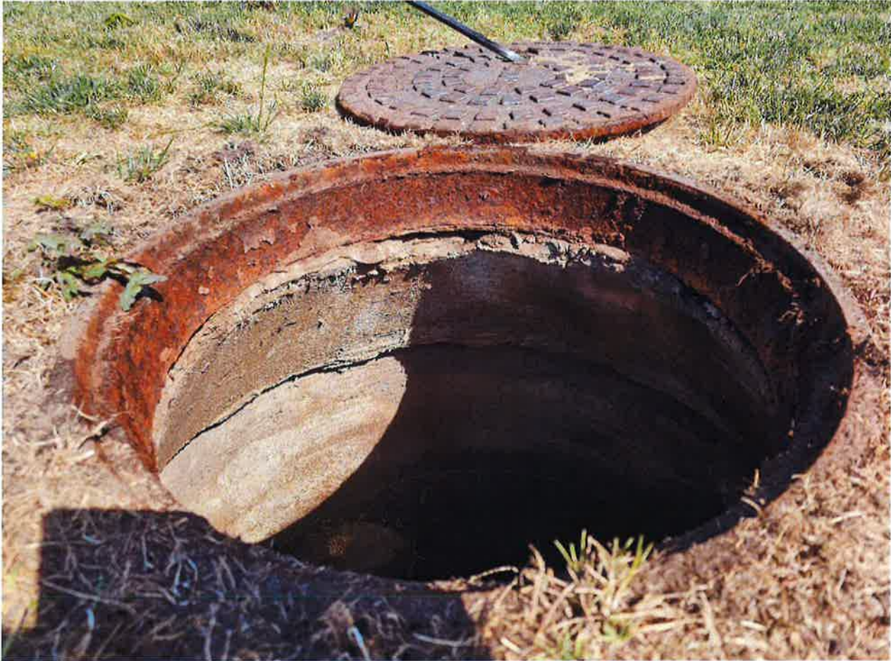
MH-4 Figure 6: Condition of MH-4.
