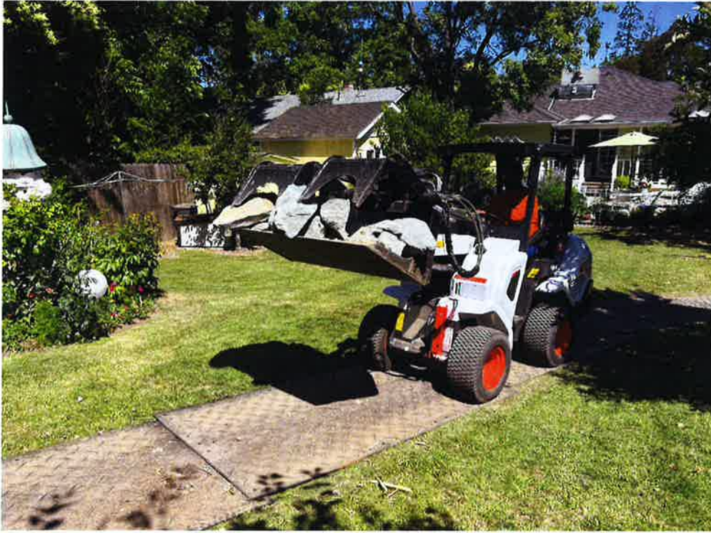
1968 Canal Drive: Methodology used to transport RSP to the waterside slope.
