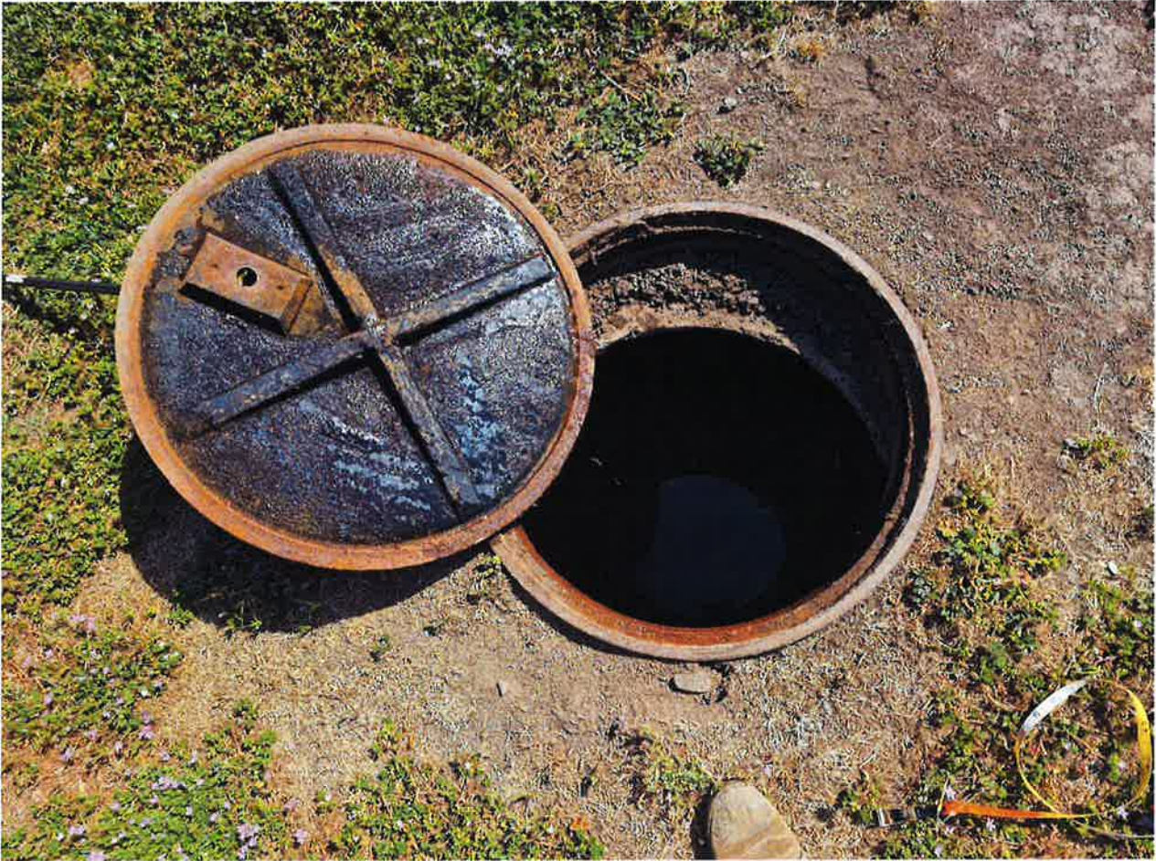
MH-2 Figure 4: Condition of MH-2.
