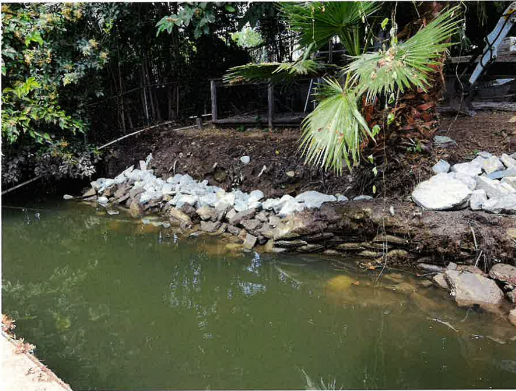
Prep and key-in at 2374 Canal Drive
