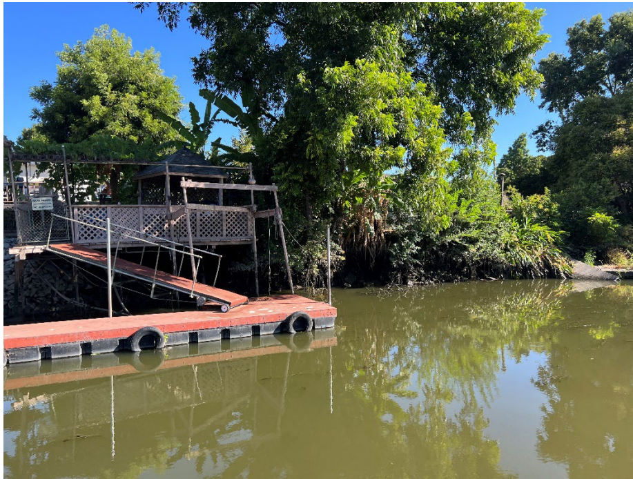
1954 Canal Drive (right side of white deck): This owner approached the RSP Contractor requesting rock on their levee slope after he had mobilized his equipment to another RSP site.
