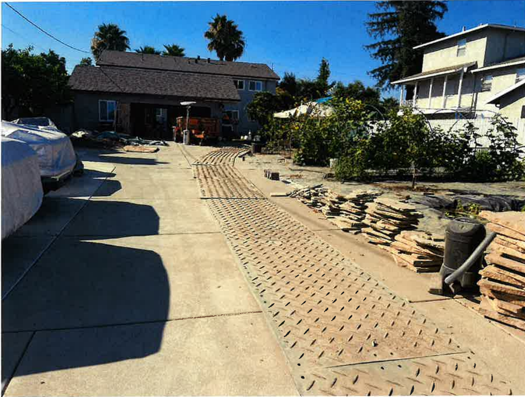
Steel plates at 2324 Canal Drive
