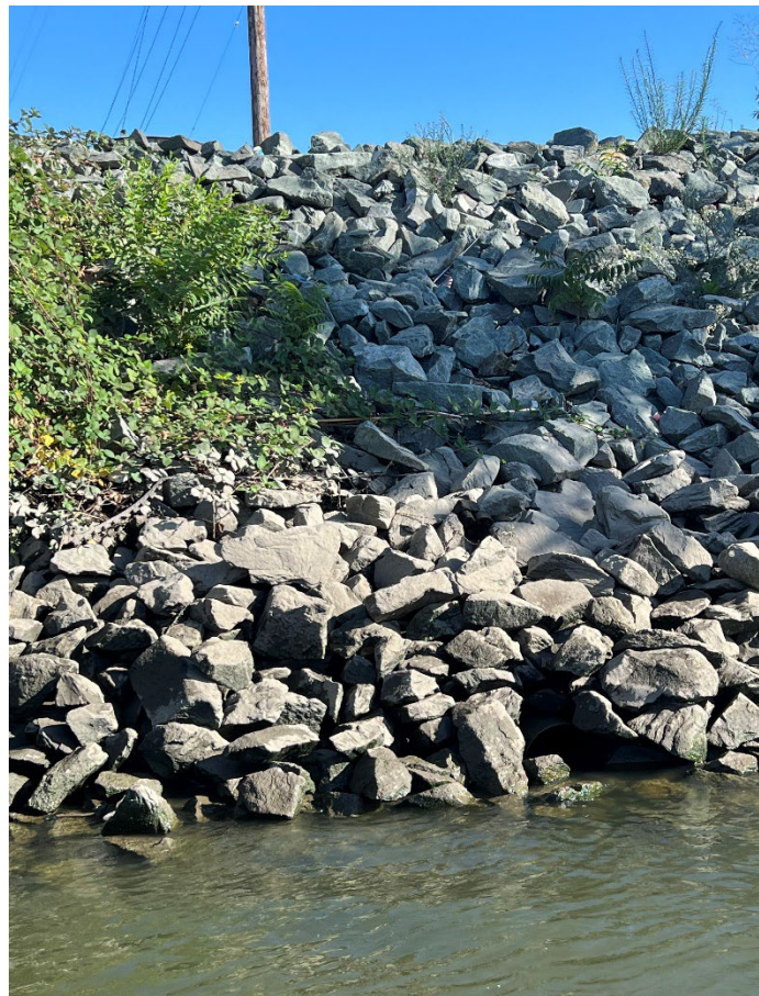
The discharge pipe (bottom) at pump sta. 4
