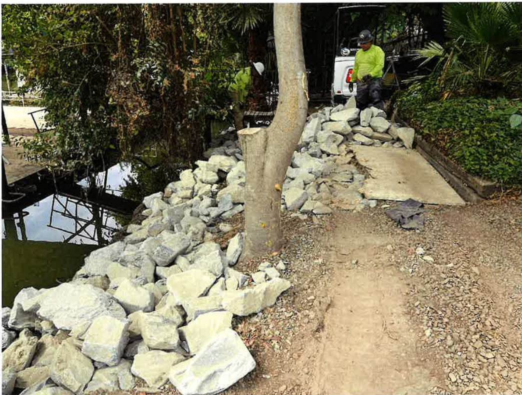
Hand placement of RSP at 2374 Canal Drive
