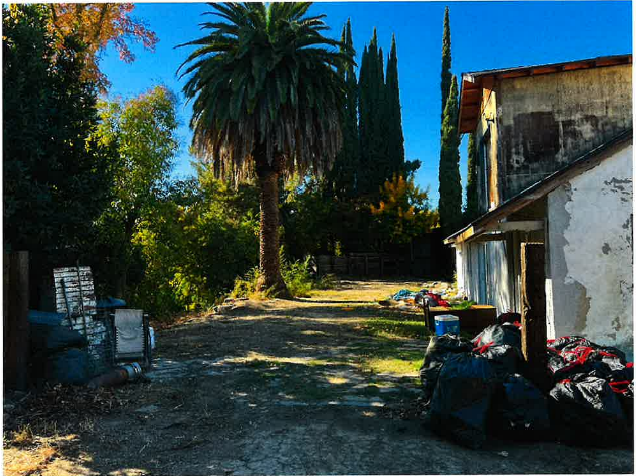
Figure 1 - Existing House and Backyard Looking West (Day 1 before prep work on 11/20/2023)
