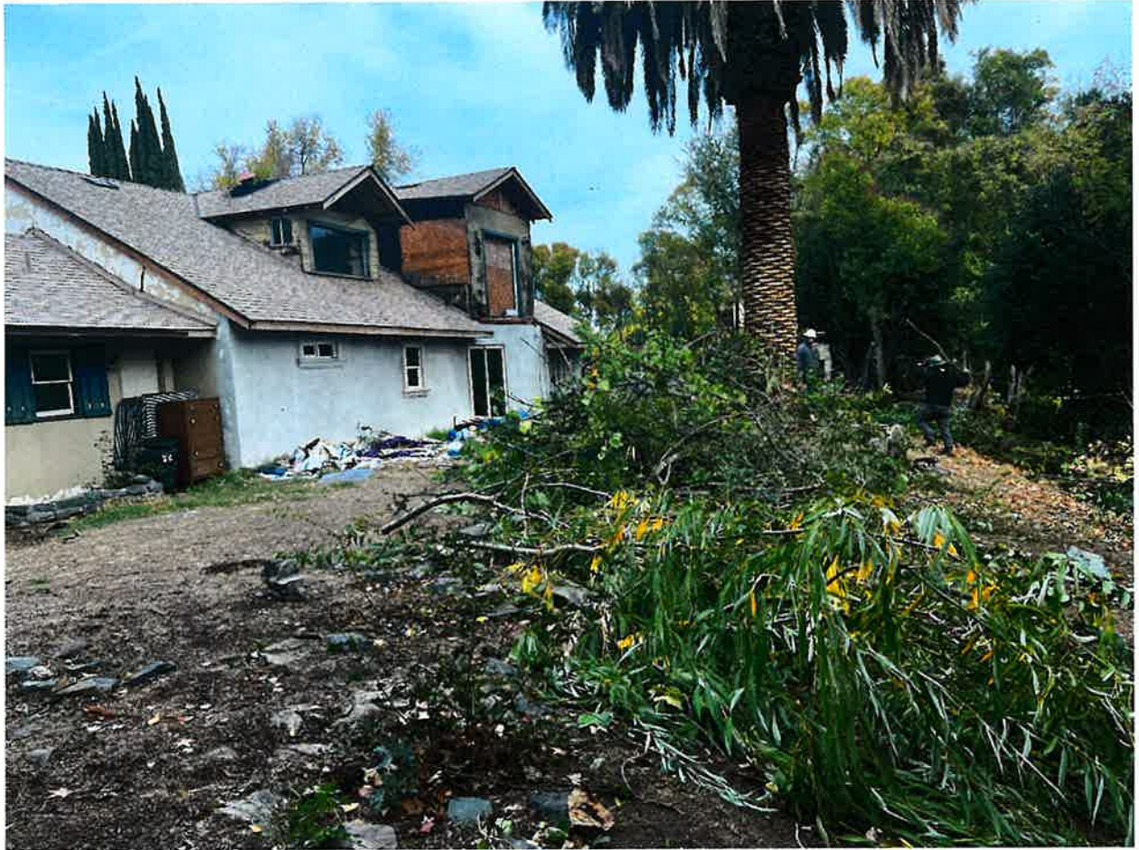
Figure 2 - House and Backyard Looking East (Day 2 of prep work on 11/21/2023)
