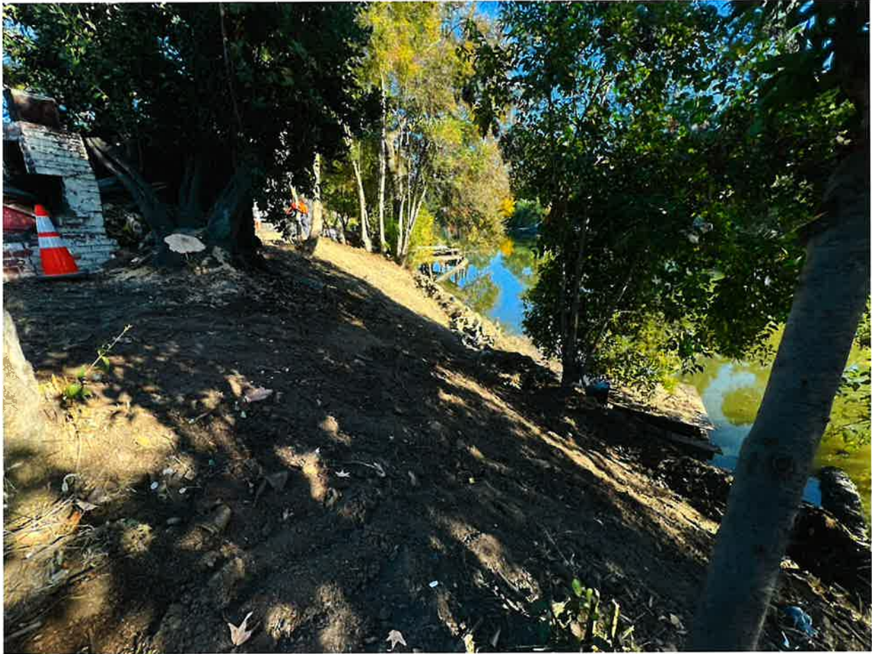
Figure 3 - Levee Slope Looking East (post-prep on 11/29/2023)
