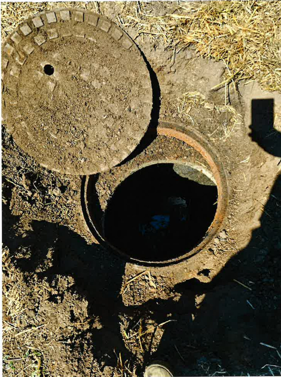
Figure 5 - Manhole 1 at HTLL
