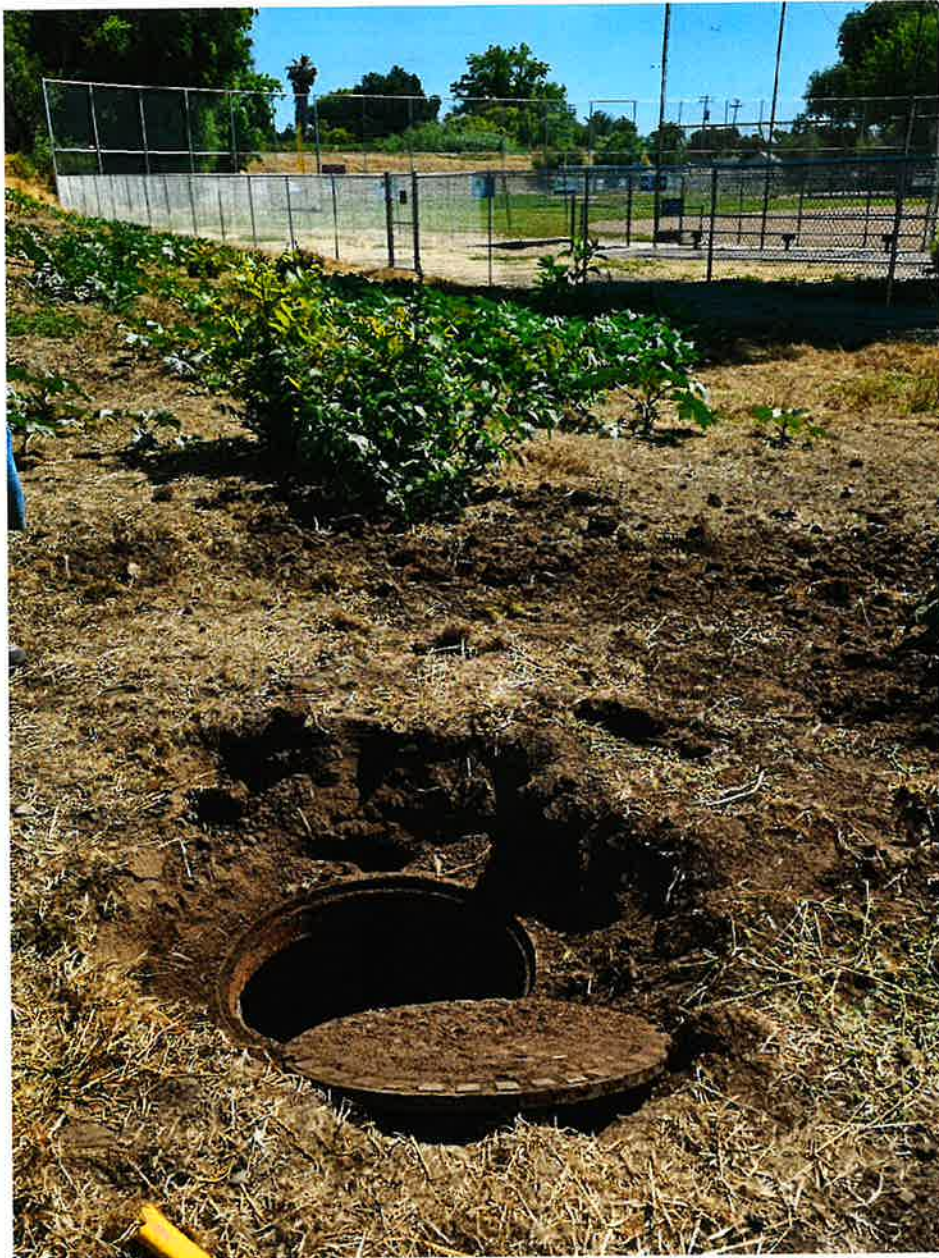
Figure 4 - Manhole 1 at HTLL
