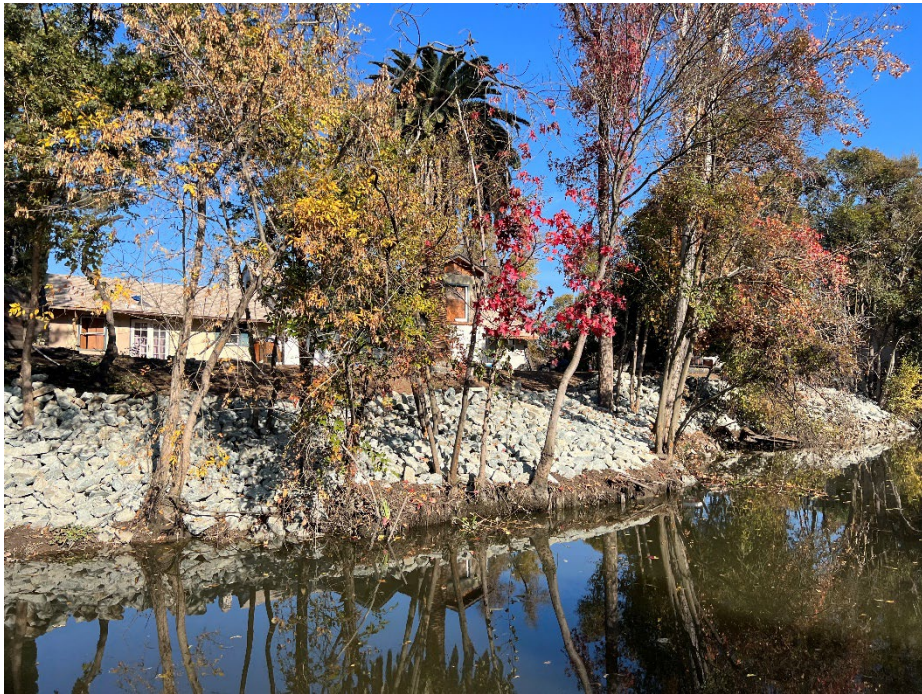
1616 S Tuxedo Ave.: RSP placement in progress.
