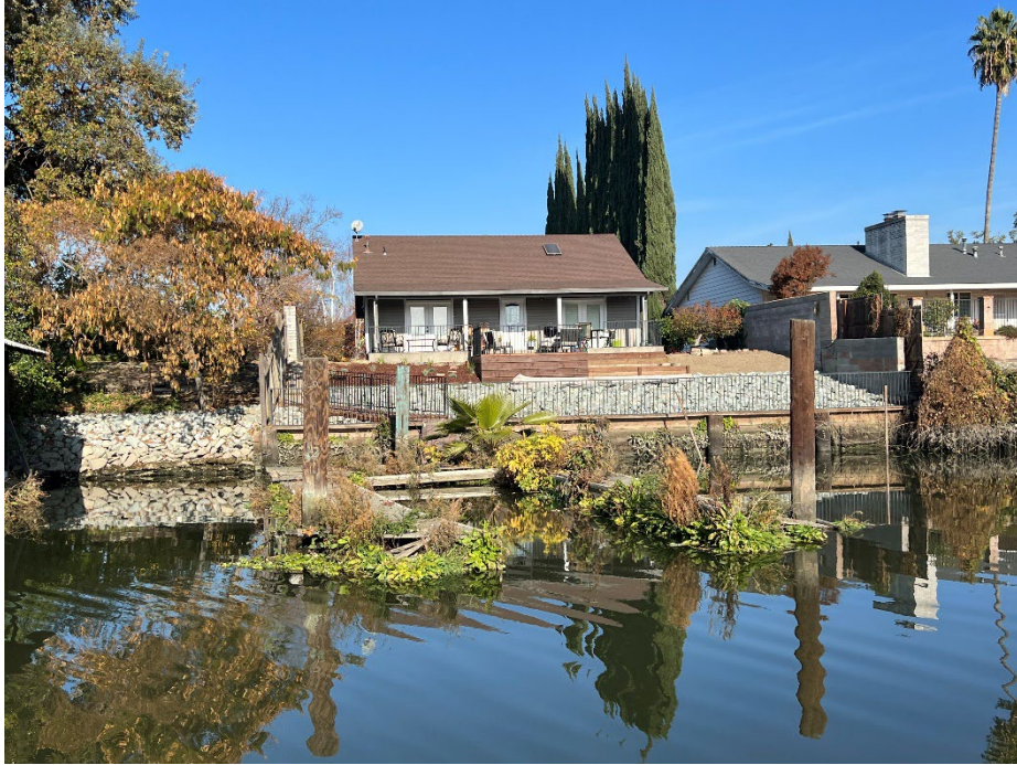
2364 Canal Dr.: Property had RSP installed earlier in the year.
