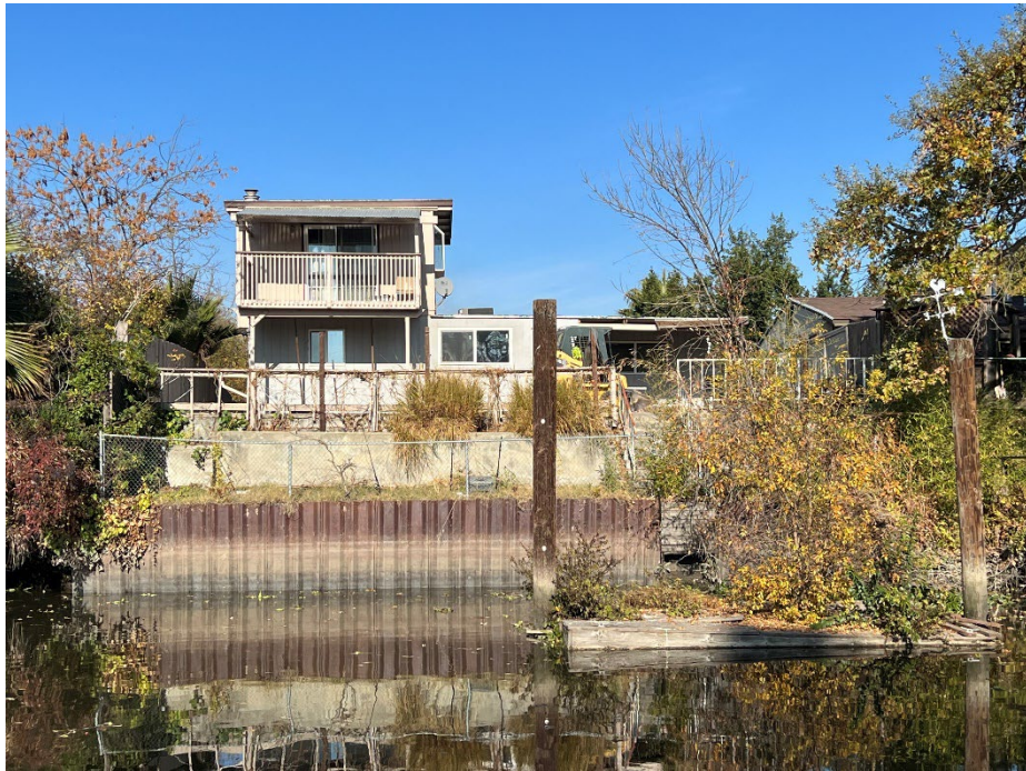
1522 S Tuxedo Ave.: Earthwork machinery is seen grading the levee crown in photo.
