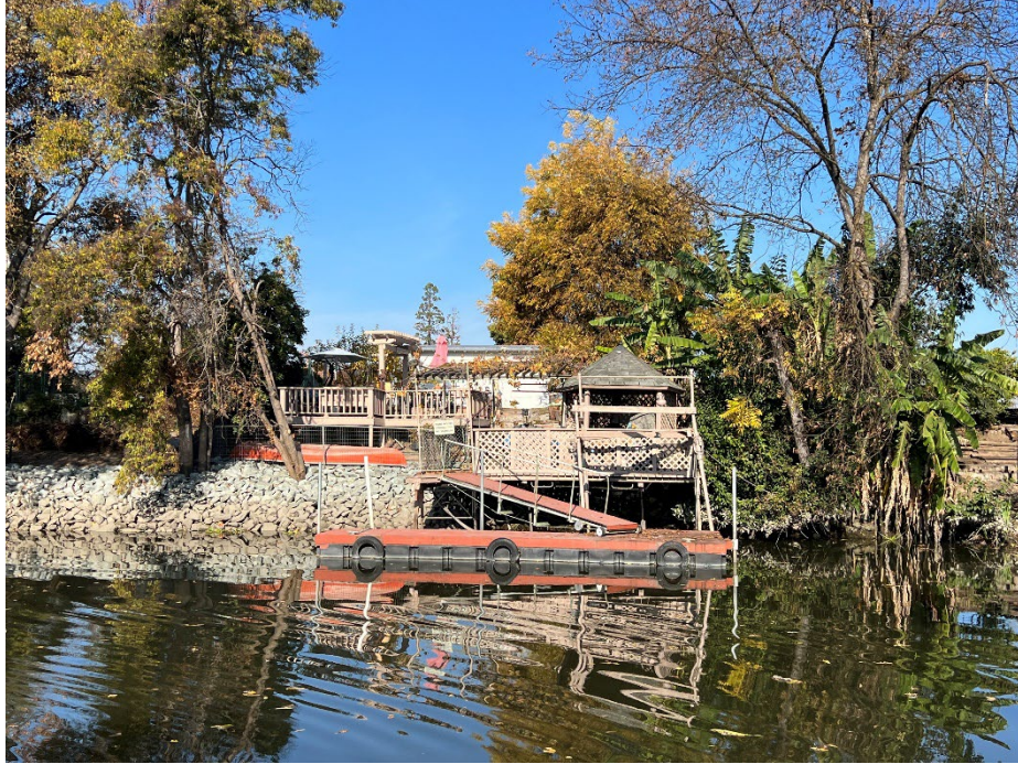
1960 Canal Dr.: A property who had RSP installed earlier in the year.
