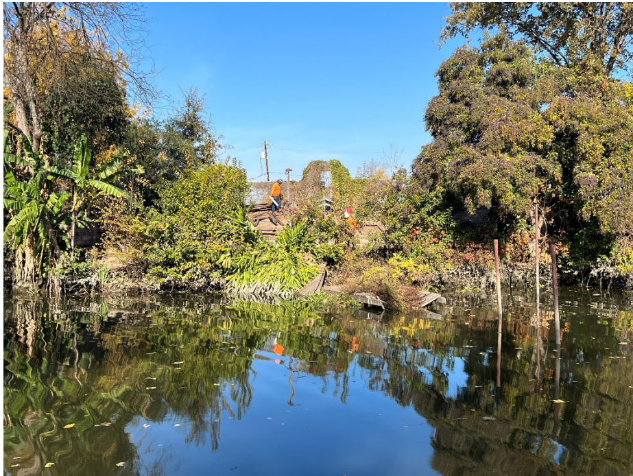
1954 Canal Dr.: Clearing of vegetation currently in progress for RSP placement.
