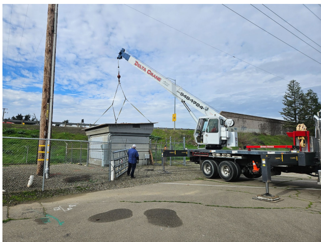
Roof of building being removed by crane
