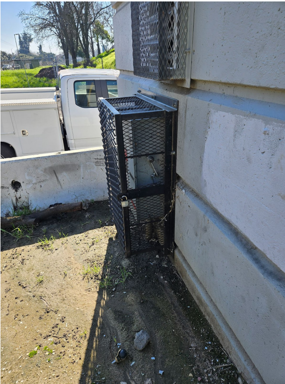
Steel grating was cut - exposing power switch- Debris piled up at station, note solar panel on roof
