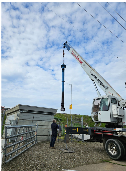
Pump being removed and set on truck
