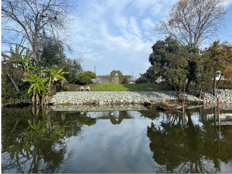
1954 Canal Drive following RSP placement: This property was an absolute disaster prior to its present state.
