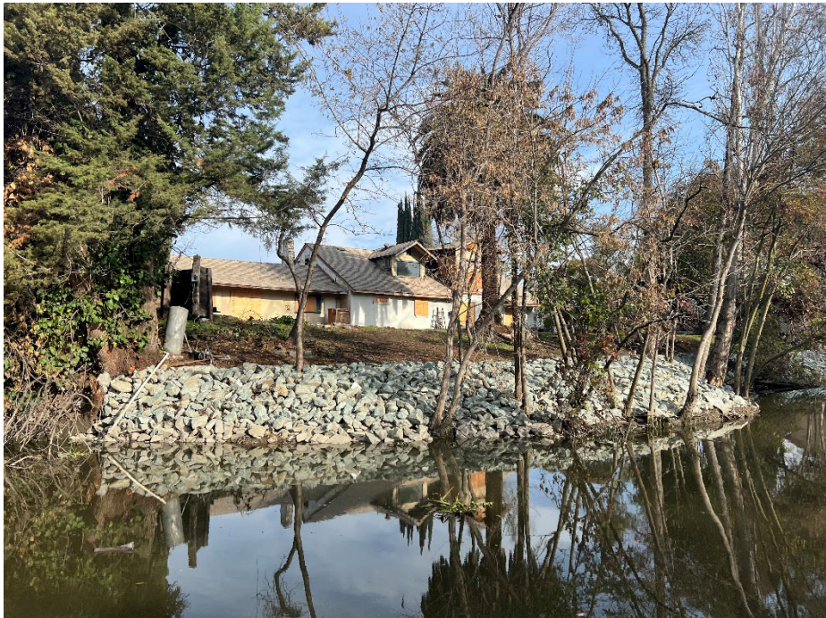
1616 S Tuxedo Ave. post-RSP placement.
