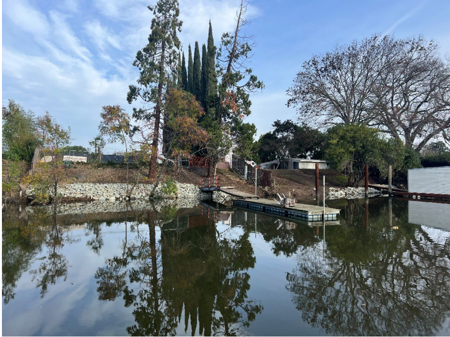
2050 and 2060 Canal Drive: RSP placement is in progress.
