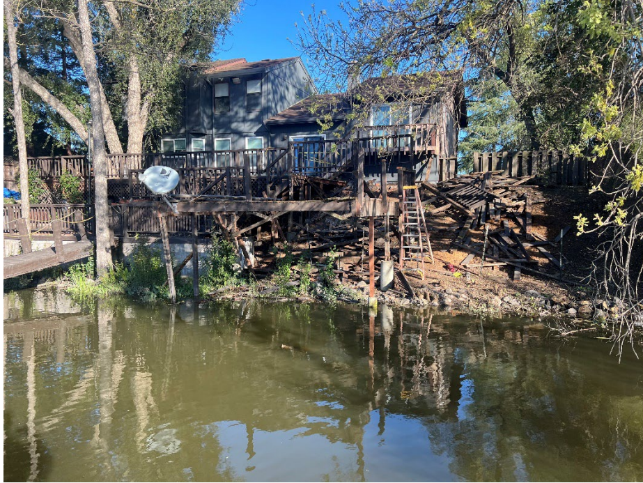
2012 Franklin Ave.: Deck demo/replacement is in progress on the levee slope.
