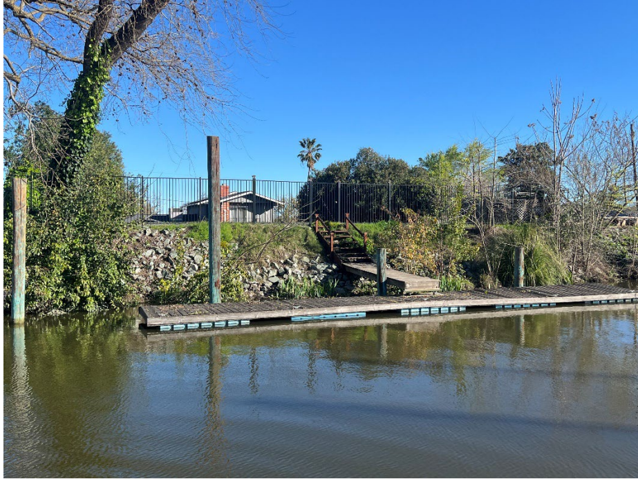
2016 Canal Drive: RSP from a past project is visible on the slope.
