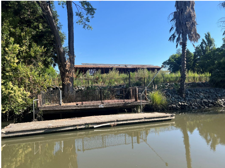
3216 Moering Ct.: No improvements on the gutted house located on the levee landside have been made in quite awhile.
