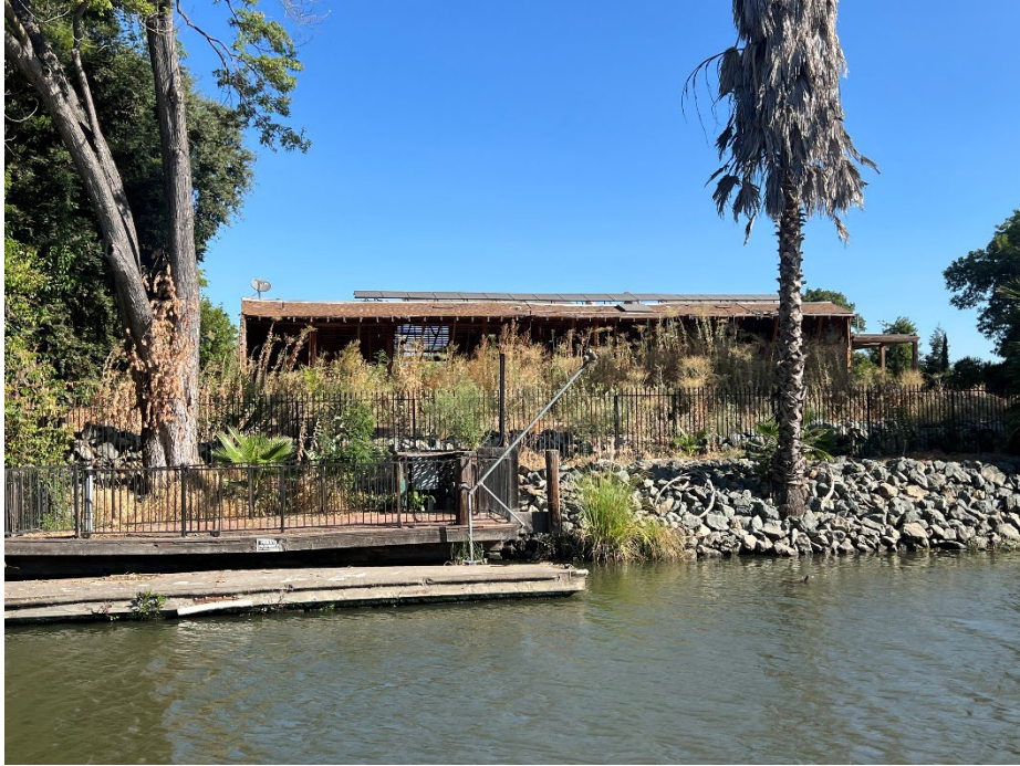
3216 Moering Ct.: Still no improvements to the gutted house.
