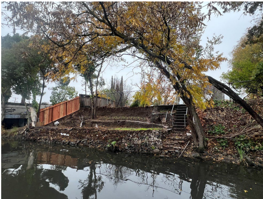
1701 Pershing Ave.: The homeless camp was removed from this property and slope modifications conducted by the property owner.
