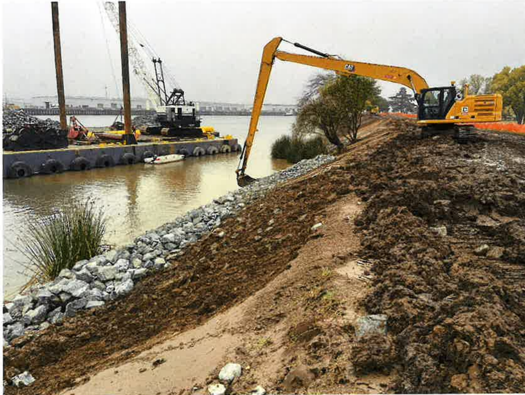
Placement of riprap.
