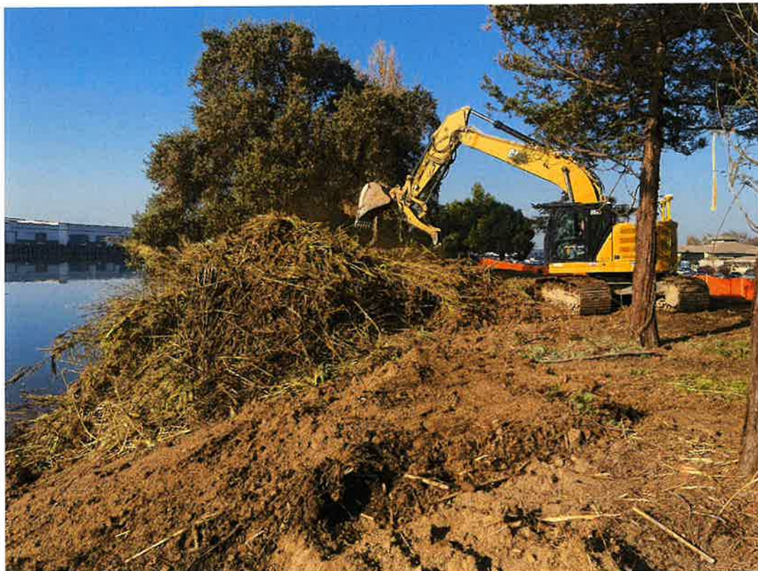
Removal of Arundo.
