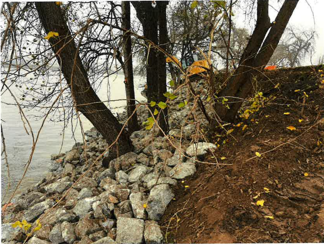
Placement of riprap around trees.
