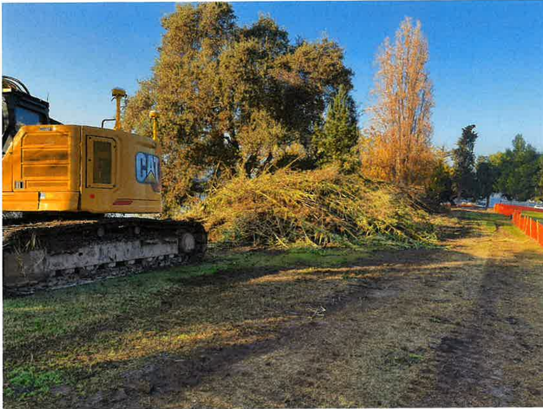
Removal of Arundo.
