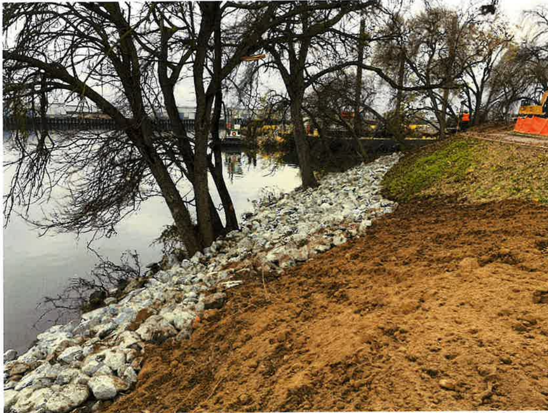
Placement of riprap around trees.
