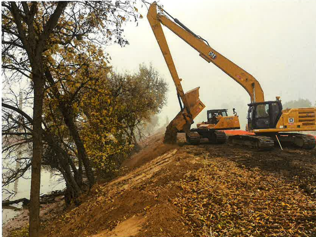
Placement of fill material.
