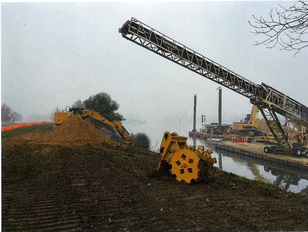
Conveyor unloading fill material.
