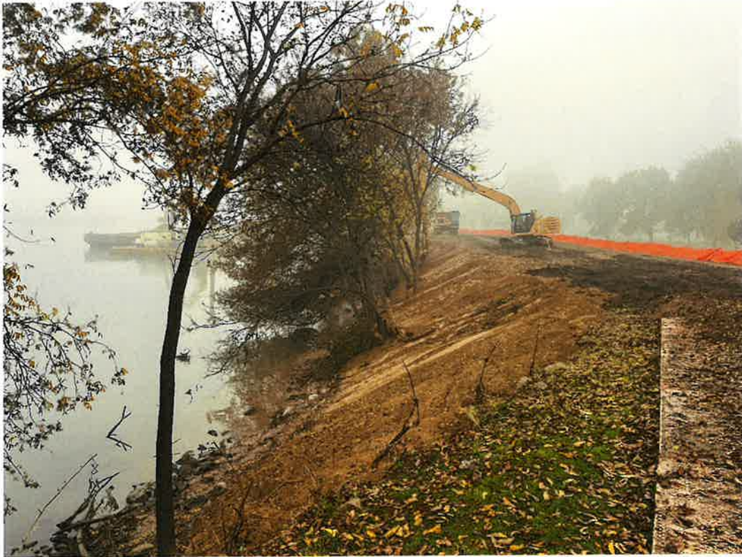
Placement of fill material.
