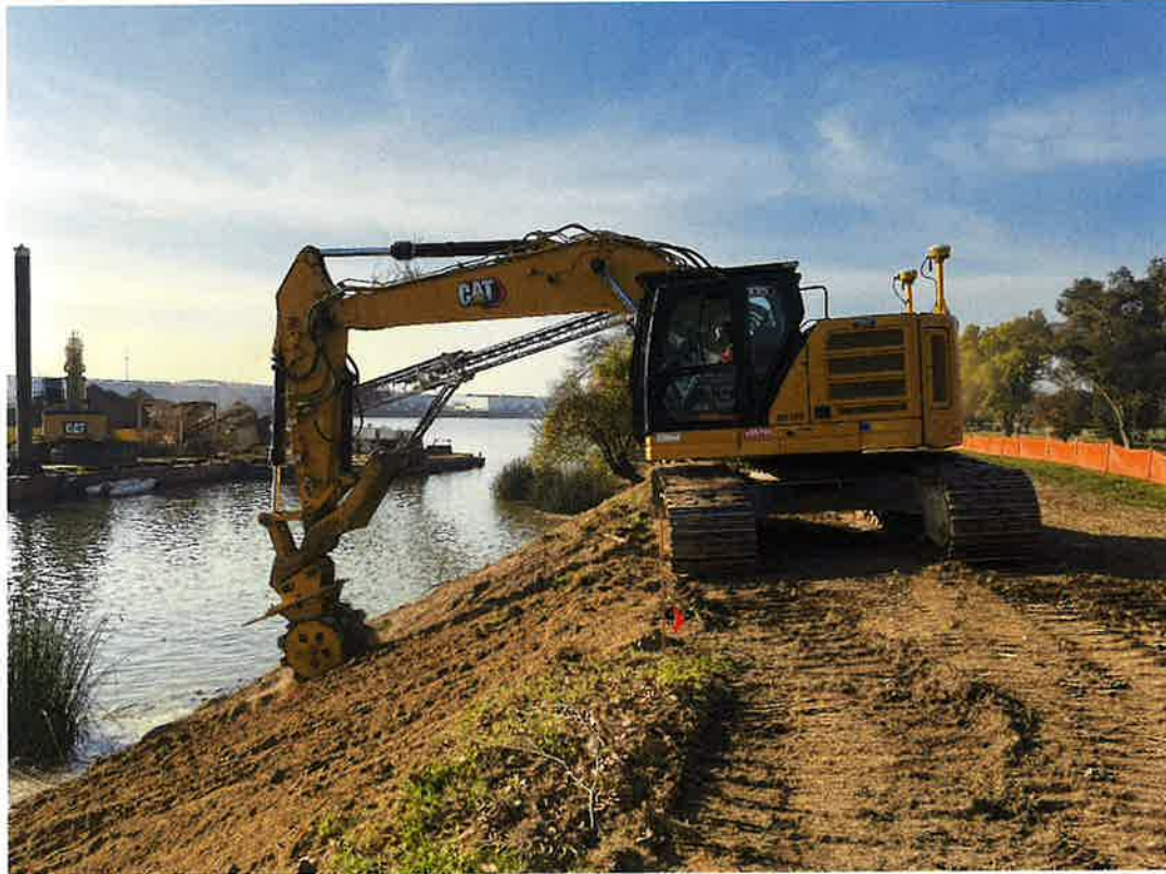
Compaction of fill material.
