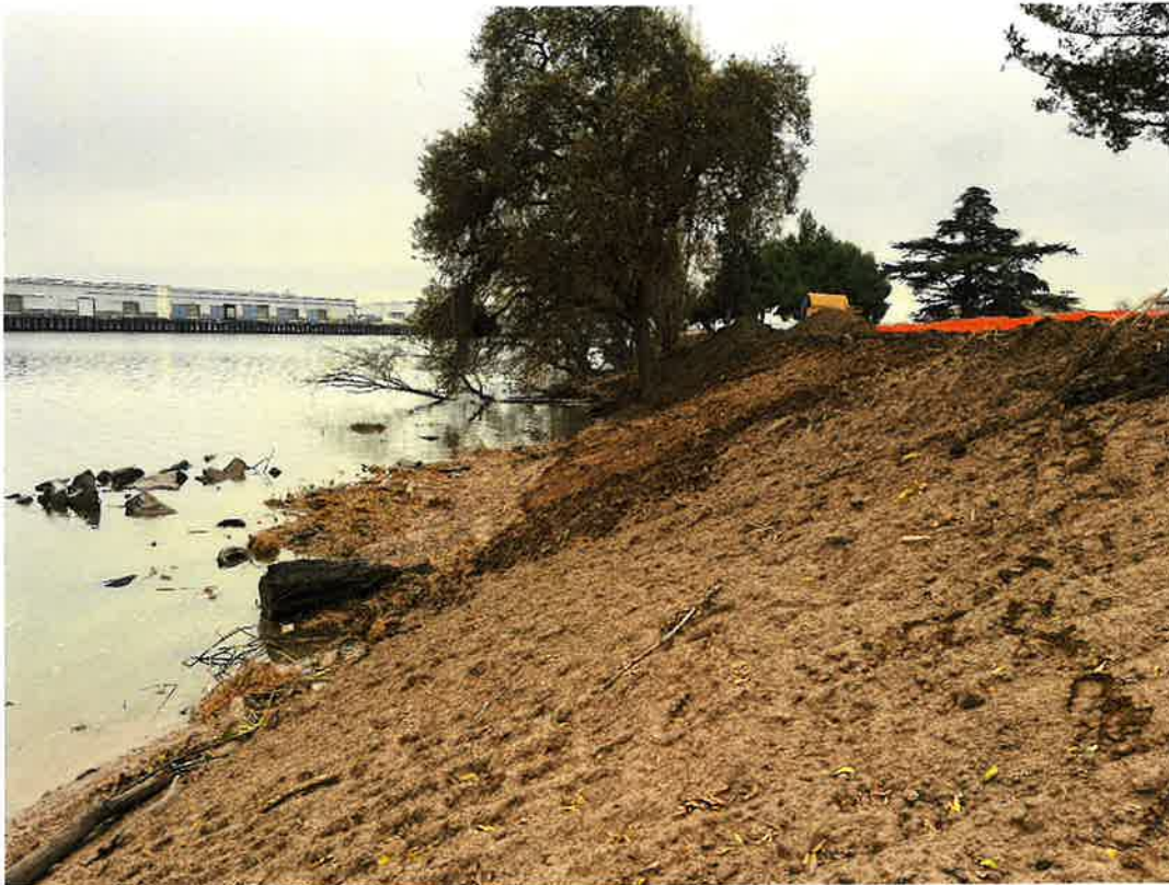
Finished slope after Arundo removal.
