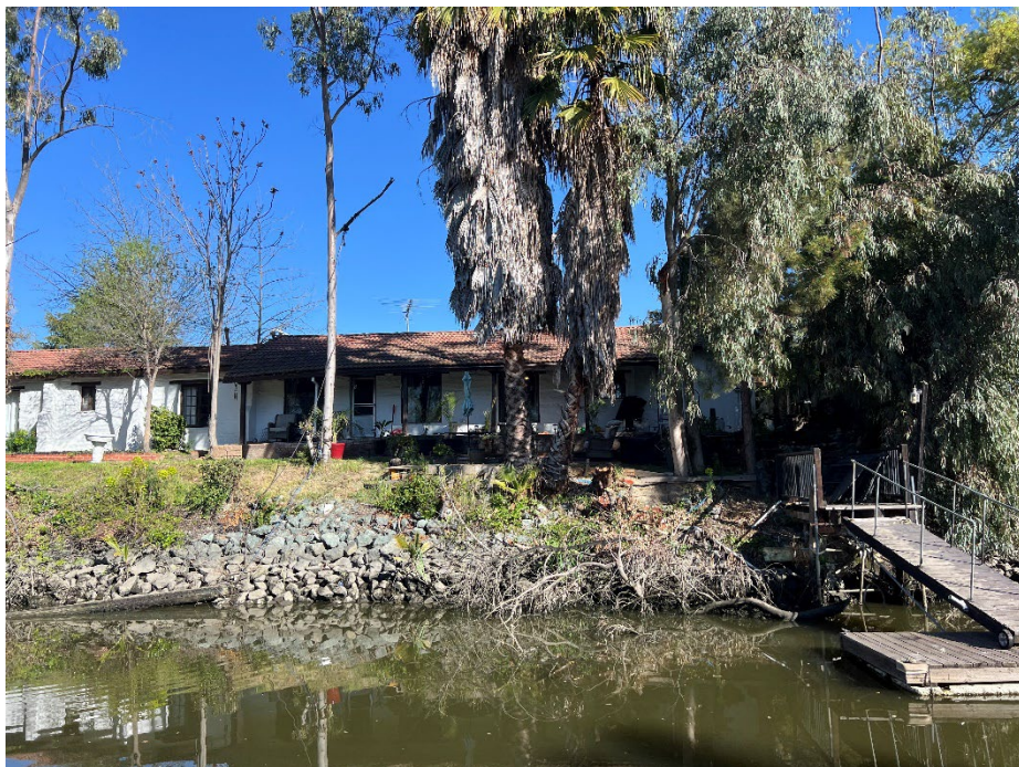
1722 W. South Tuxedo Ave.: Old rock slipping down the waterside slope
