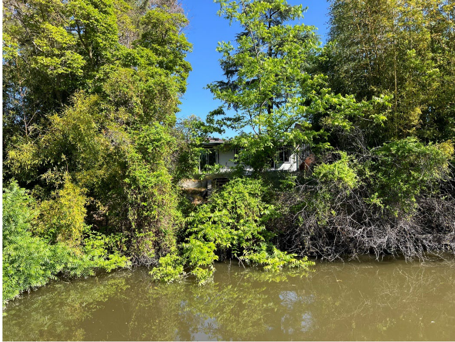
1448 W. South Tuxedo Ave.: Dense vegetative overgrowth on the levee slope.
