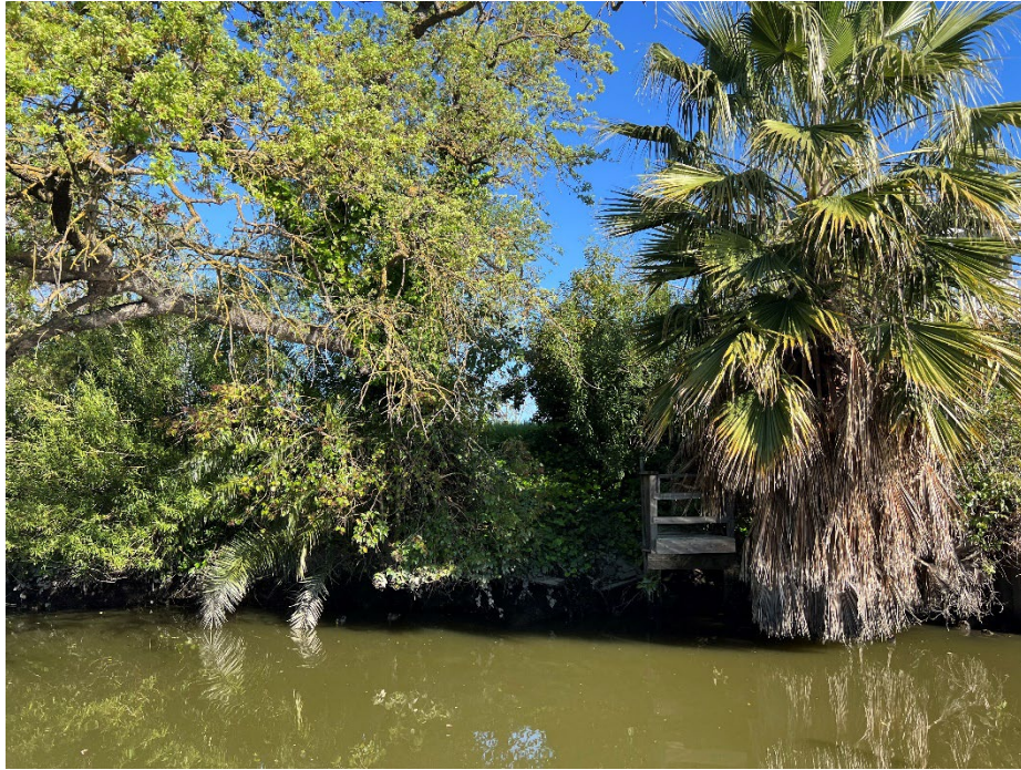
1534 W. South Tuxedo Ave.: Yet more dense vegetation on the levee slope making inspection impossible.
