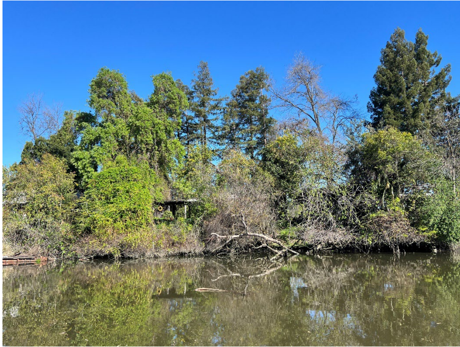
2024 Idaho Ave.: Dense waterside slope vegetation renders the levee impossible to inspect.
