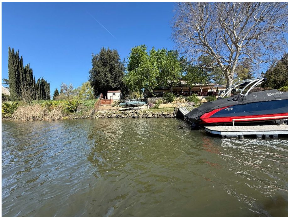
2015 Moering Rd: Wants a small section of RSP placed to the left of dock in photo.
