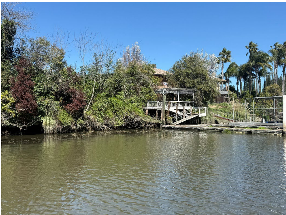
2468 Canal Drive: Property owner initially wanted RSP, then refused, then decided he wanted RSP beneath his dock because he didn't want any vegetation removed or trimmed.
