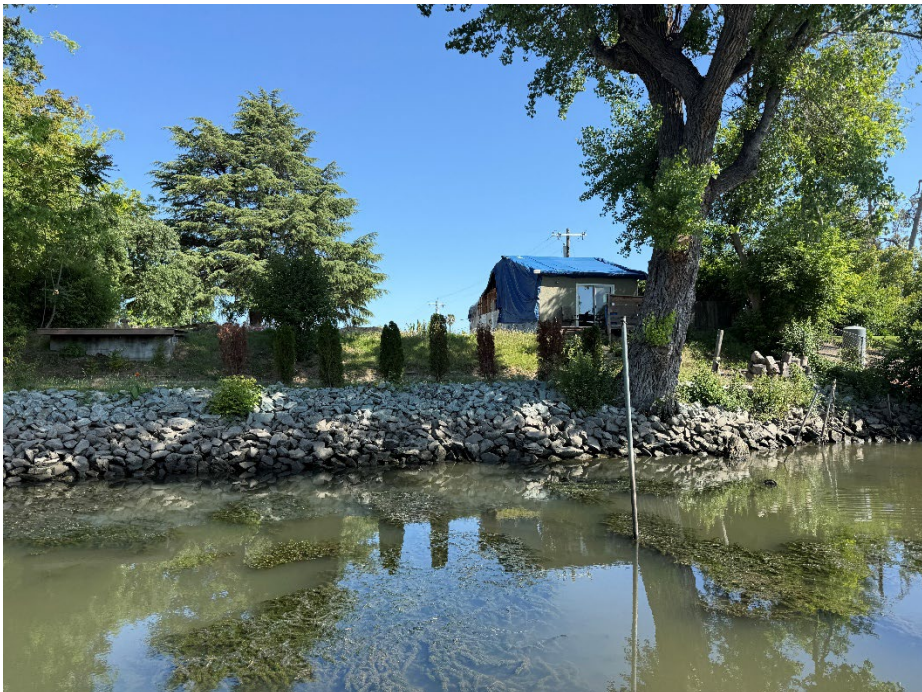
2000 Carlton Ave: This property received RSP a few years ago and the owner is in the process of remodeling the house and has planted trees on the levee waterside bench.
