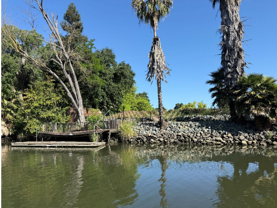
3216 Moering Ct: The dock at this property has fallen further into disrepair and the house has been demolished.
