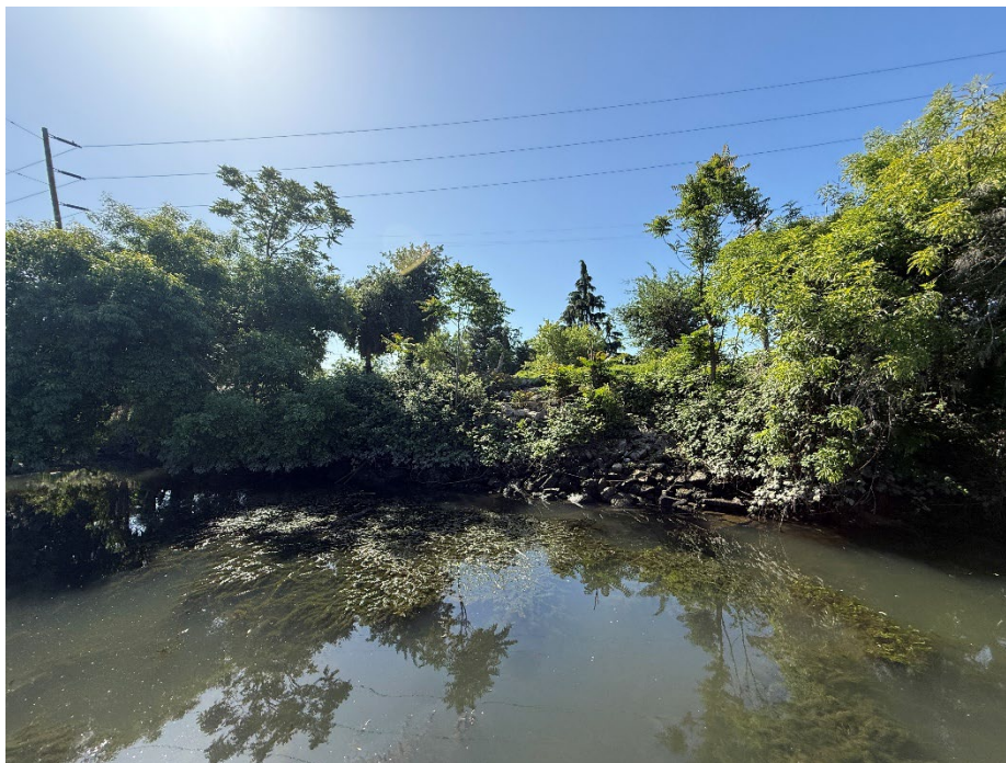
Sta. 58+00: An abandoned homeless shelter hides in the bushes along the waterside slope.
