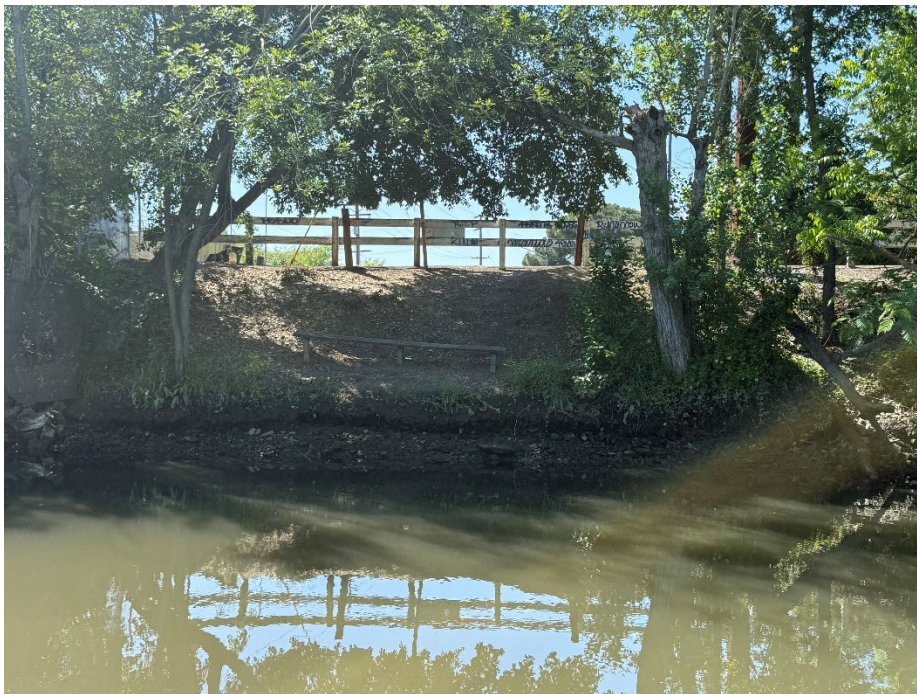
Sta. 19+00 at the end of Buena Vista Drive.
